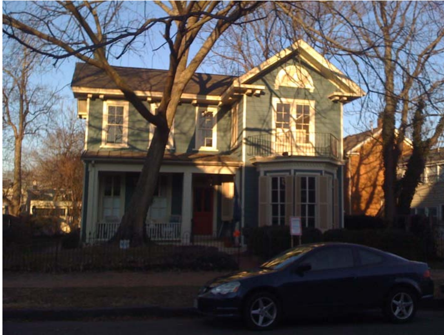
Figure 1: Front Elevation of Dwelling
