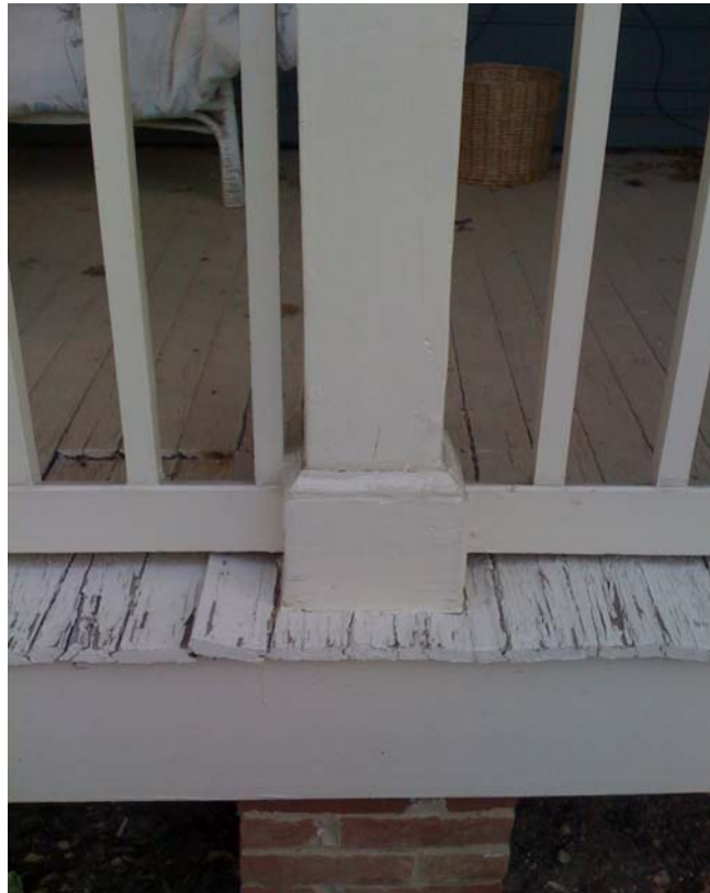
Figure 8: Detail View of Porch Post
