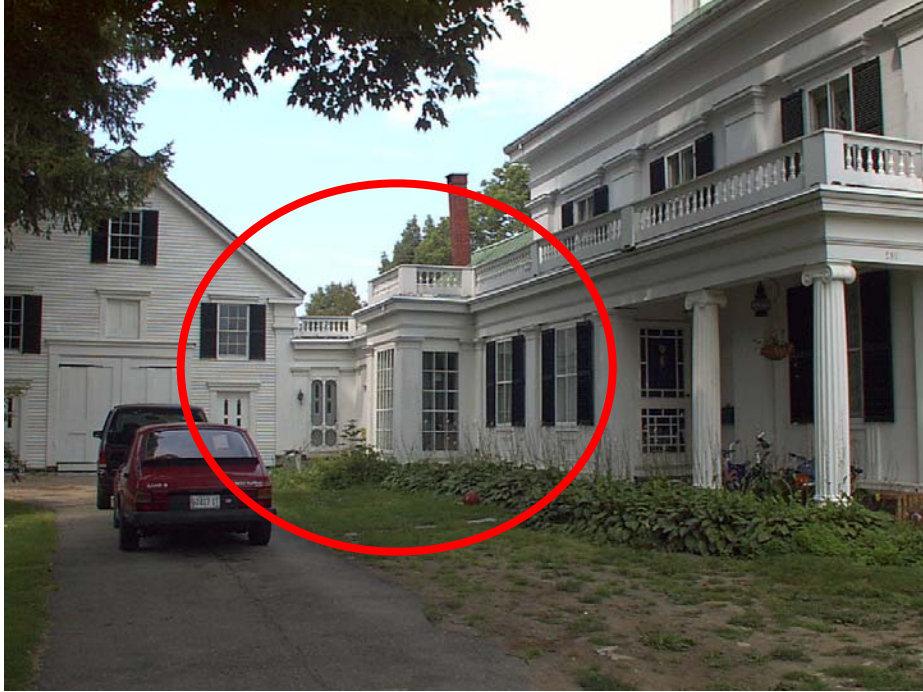
Figure 17: Example of a Glass “Hyphen” Form Attaching an Outbuilding to the Main House Note: The two massings still continue to read as two separate units.
