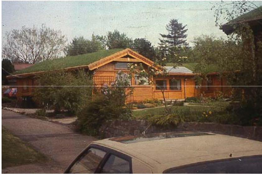
Figure 20: Example of a Solid Color “Living Roof” Mounted to a Gable Roof Form
