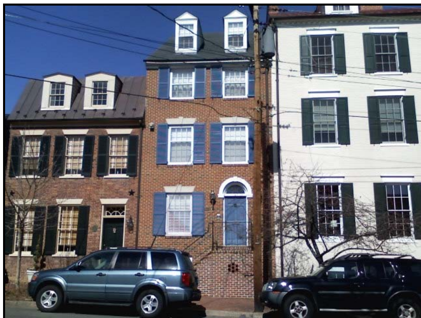
Figure 1 Photograph of Front Façade
