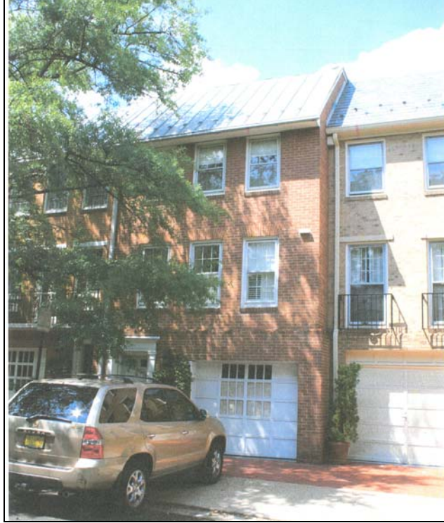
Figure 2. Front (south) elevation.
