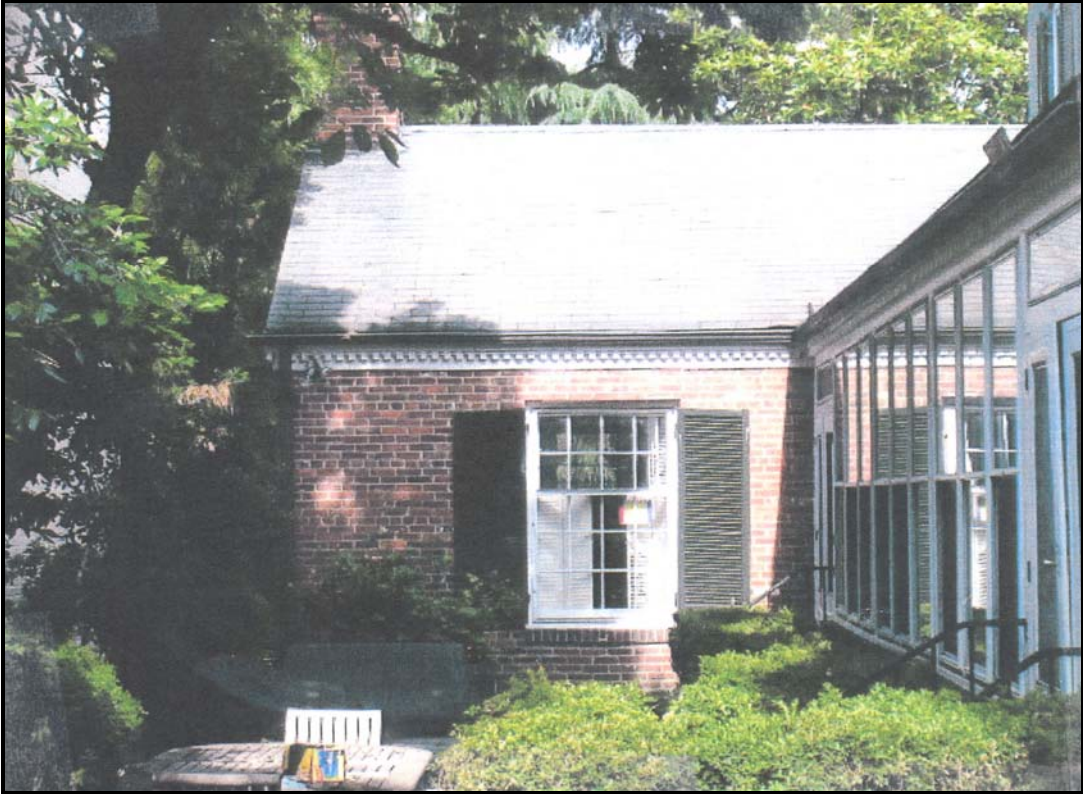
Figure 4: East Elevation of 1950s Addition
