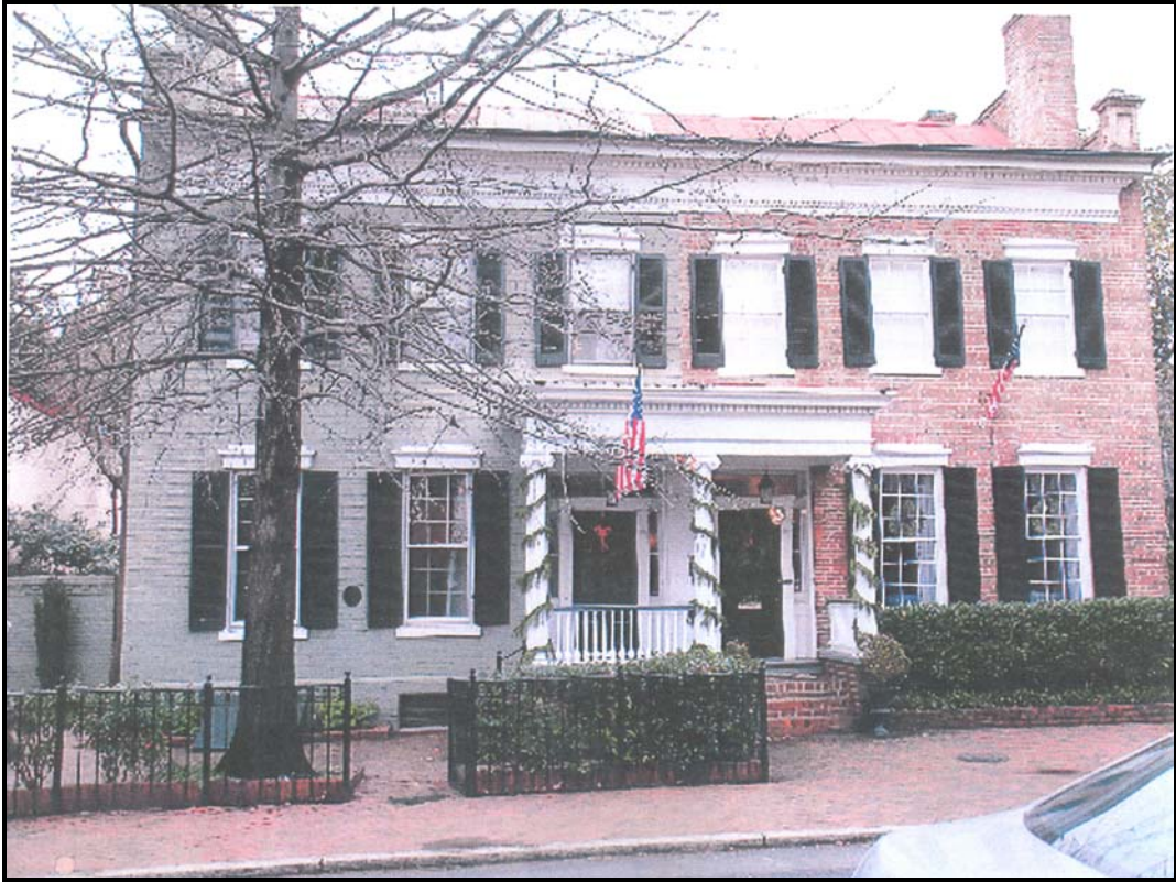
Figure 2: Front (East) Elevation
