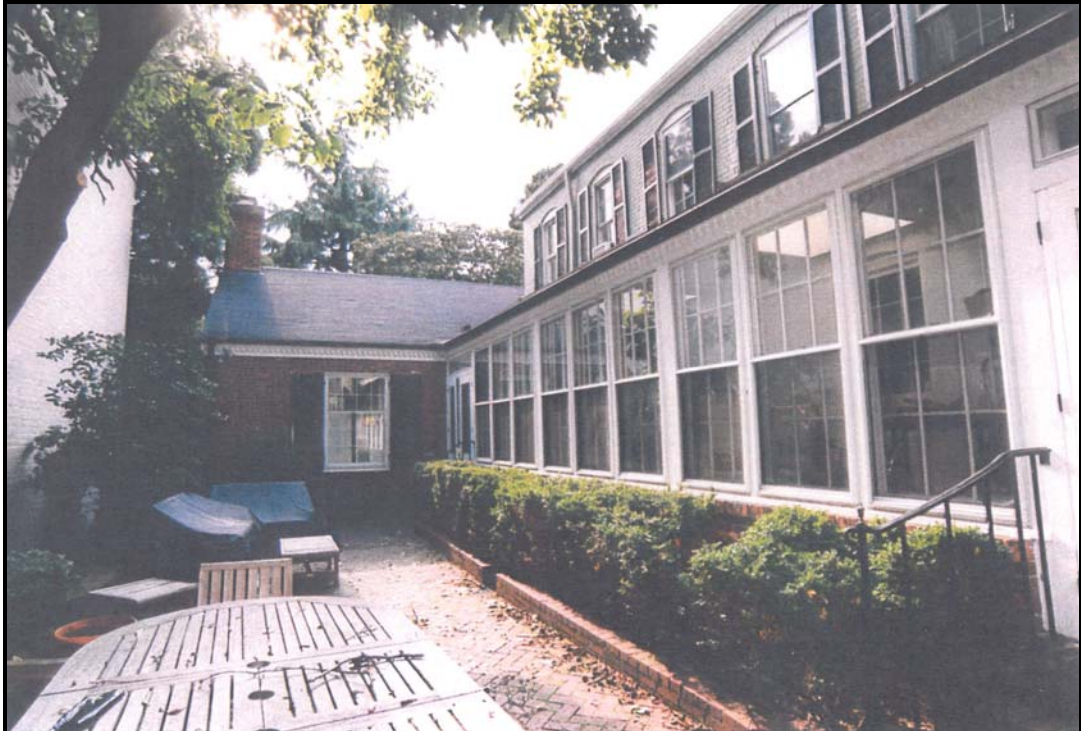
Figure 5: Existing Interior Garden and South Elevation of Main House
