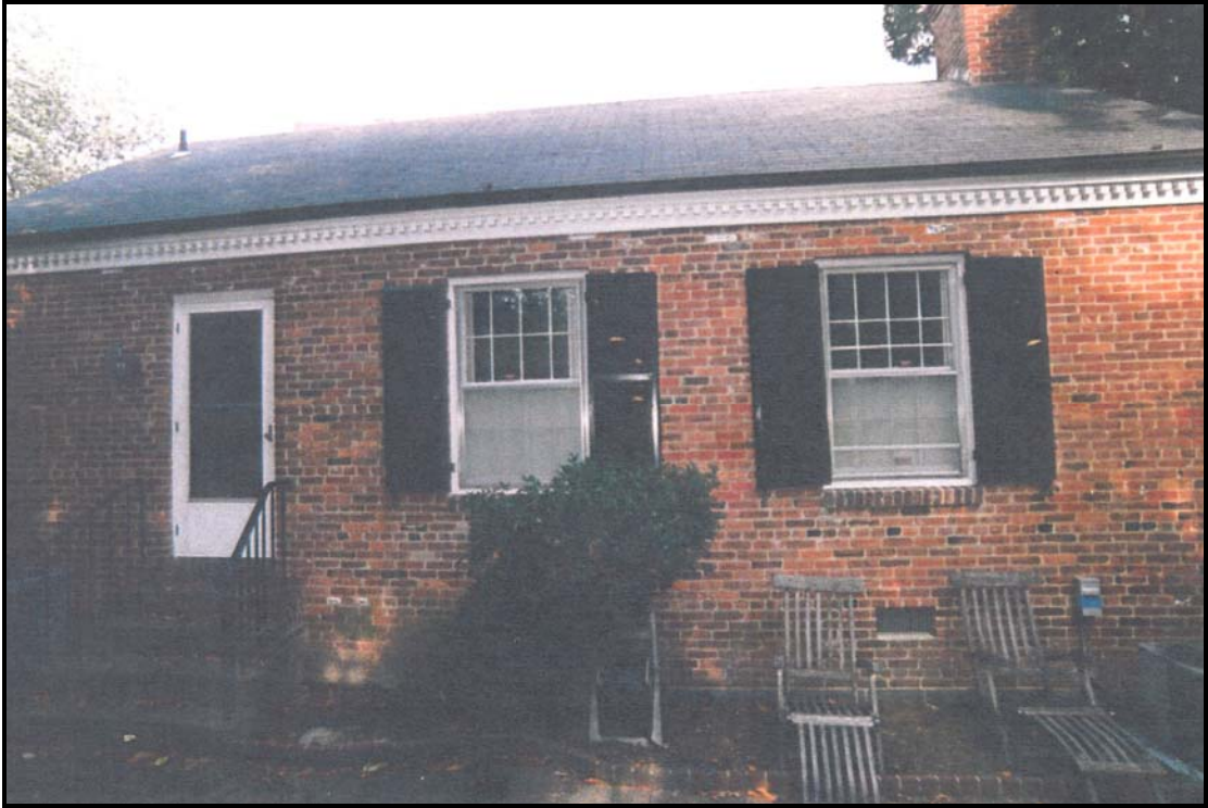
Figure 6: Rear (West) Elevation of 1950s Addition
