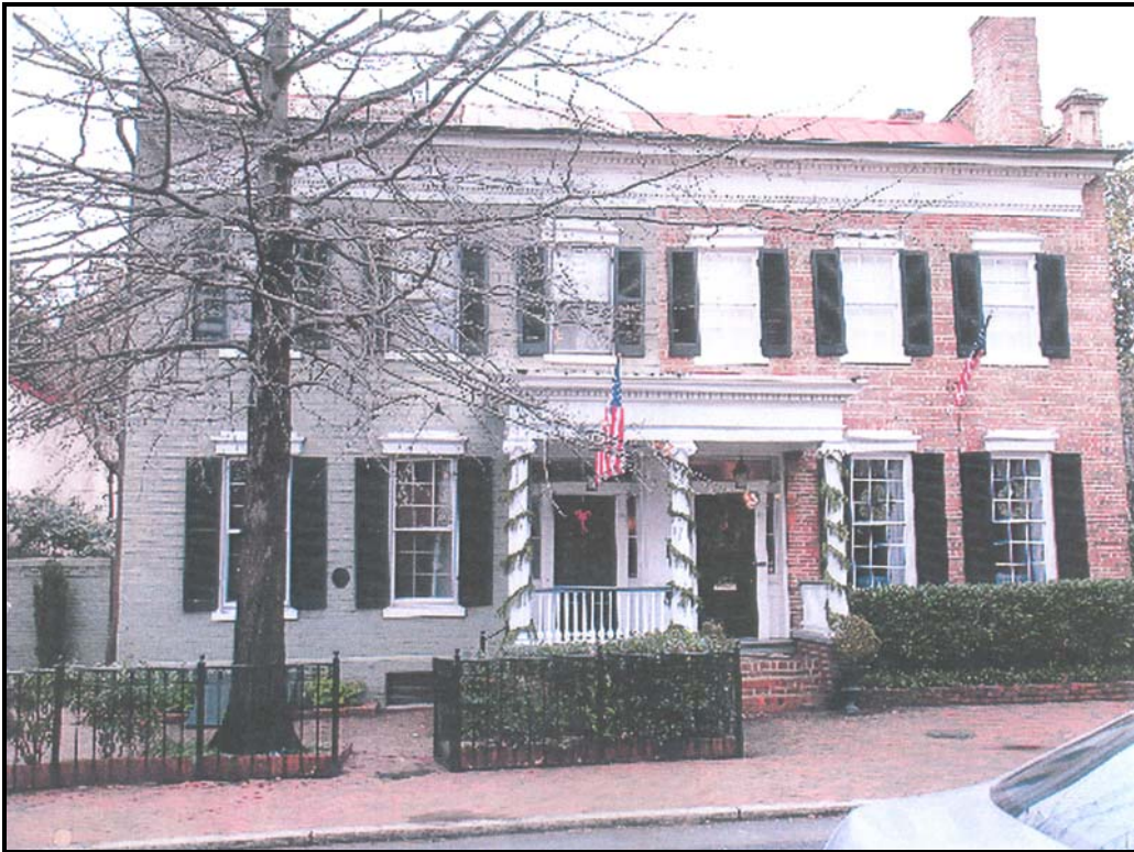
Figure 2: Existing Front/East Elevation
