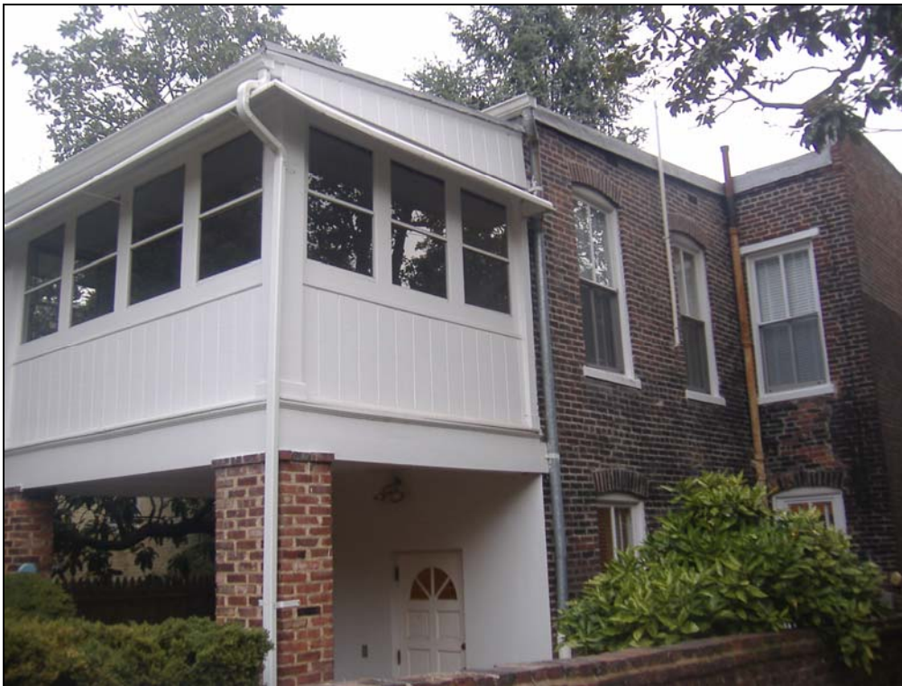
Figure 3. Rear (west) and side (south) elevations, including existing porch to be demolished.
