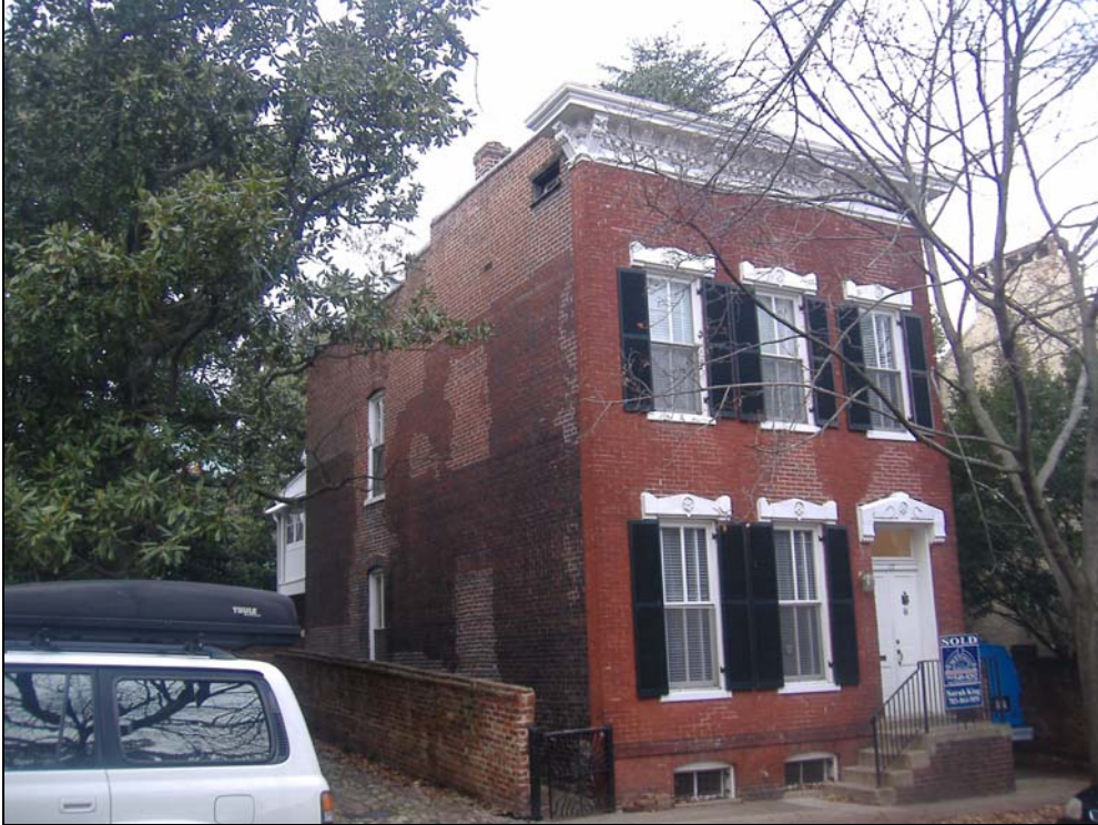
Figure 2. Front (east) and side (south) elevations, 117 South Lee Street.
