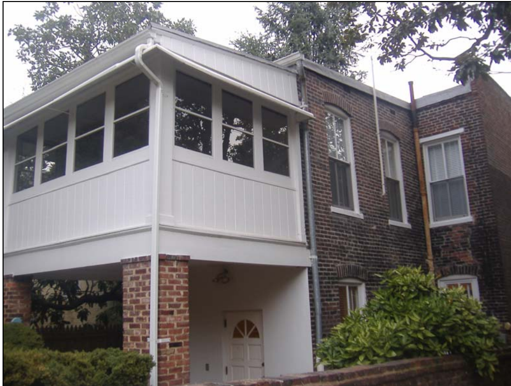
Figure 3. Rear (west) and side (south) elevations, including existing porch to be demolished.
