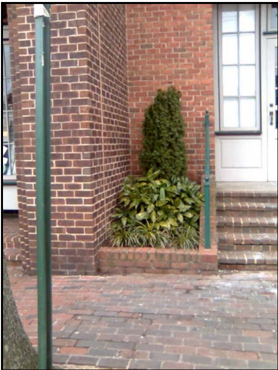
Figure 6 View of location for proposed lift.
