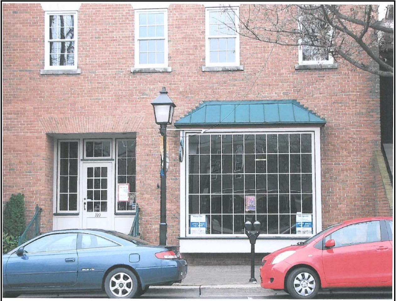
Figure 1: Photo showing existing retail storefront
