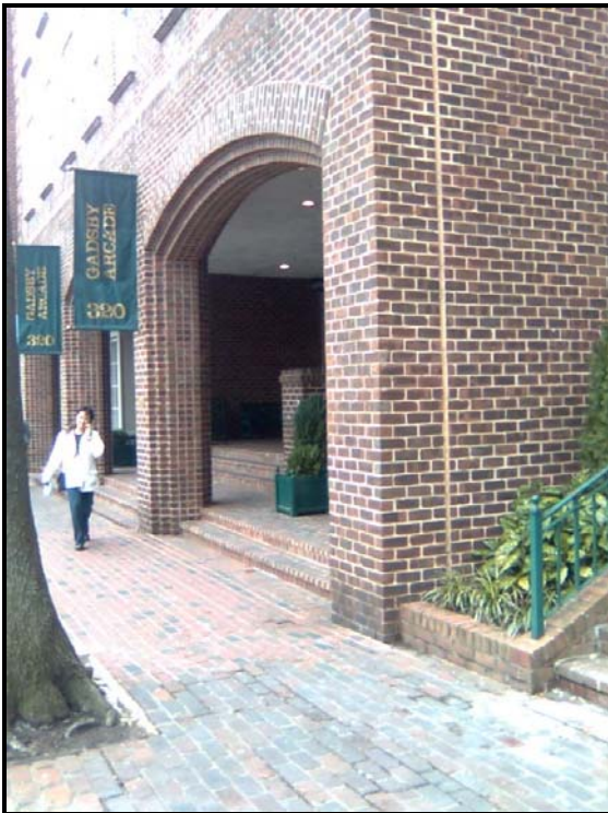
Figure 4 View of edge of tree well adjacent to current stoop.
