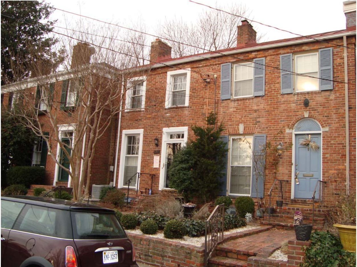
Figure 6: View of Front Elevations of Subject Property and Flanking Townhouses
