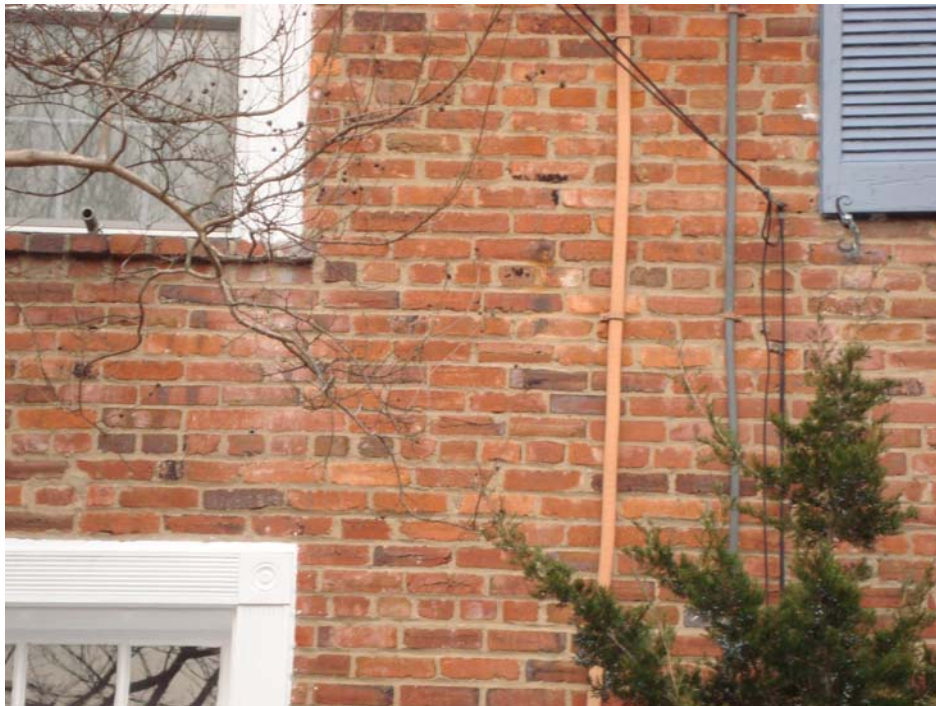
Figure 9: View of Existing Elevation's "Common Bond" Brickwork
