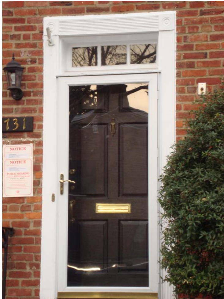
Figure 7: View of Existing Trim Detail on Front Façade
