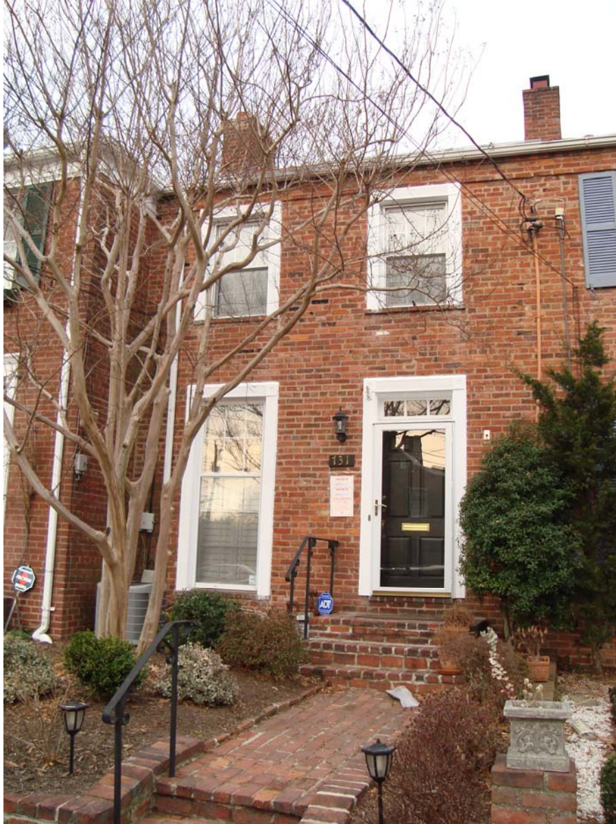
Figure 5: Front Elevation of Subject Property
