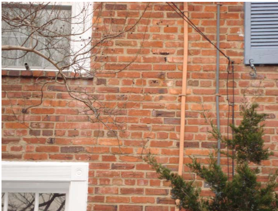
Figure 9: View of Existing Elevation's "Common Bond" Brickwork
