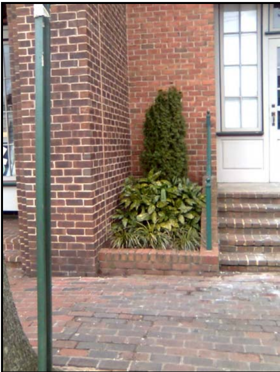
Figure 6 View of location for proposed lift.
