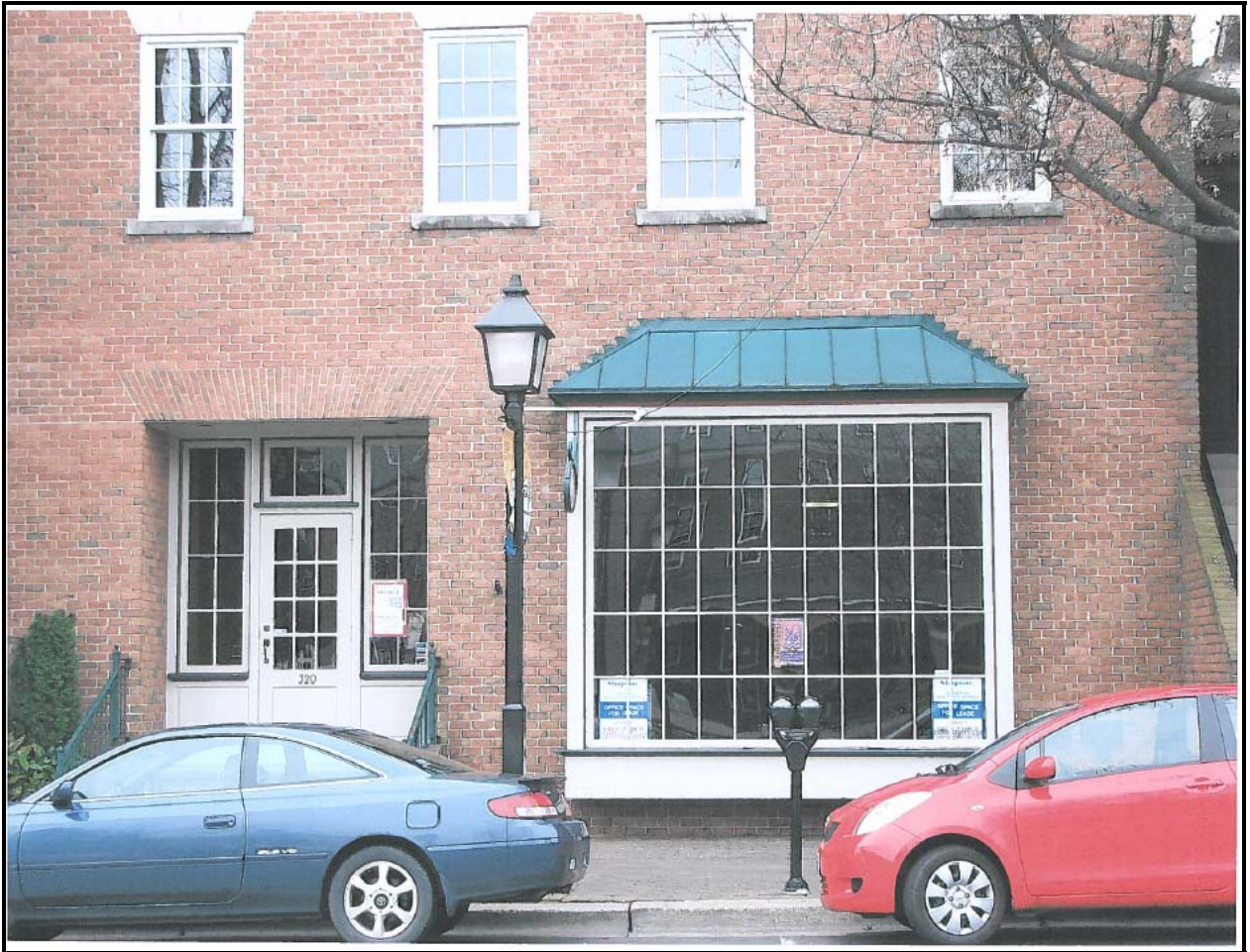
Figure 1: Photo showing existing retail storefront
