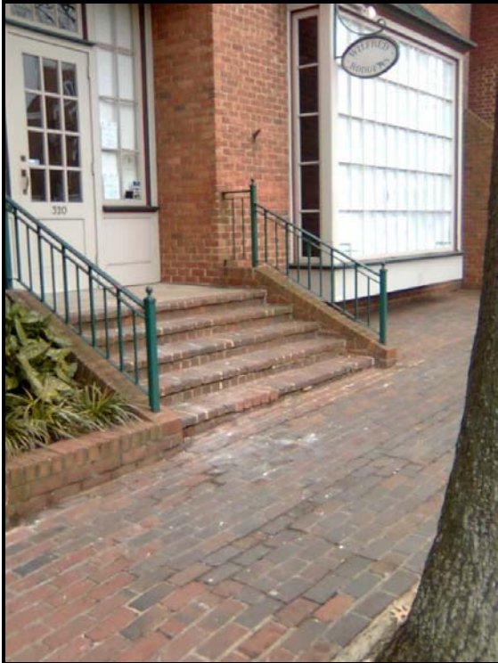
Figure 3 View of Existing Stoop looking West on King Street
