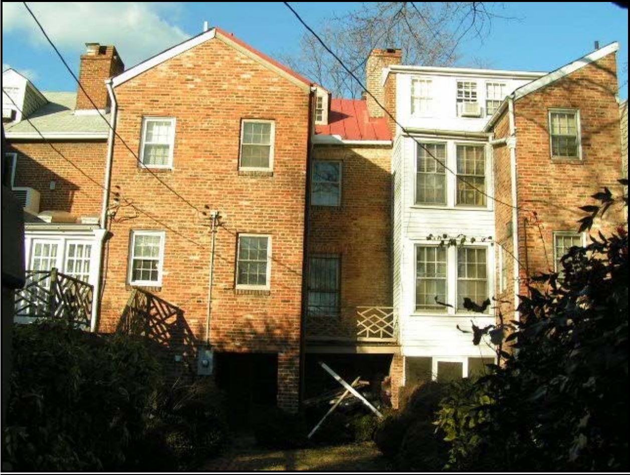
Figure 3: Rear of 1110 Prince Street
