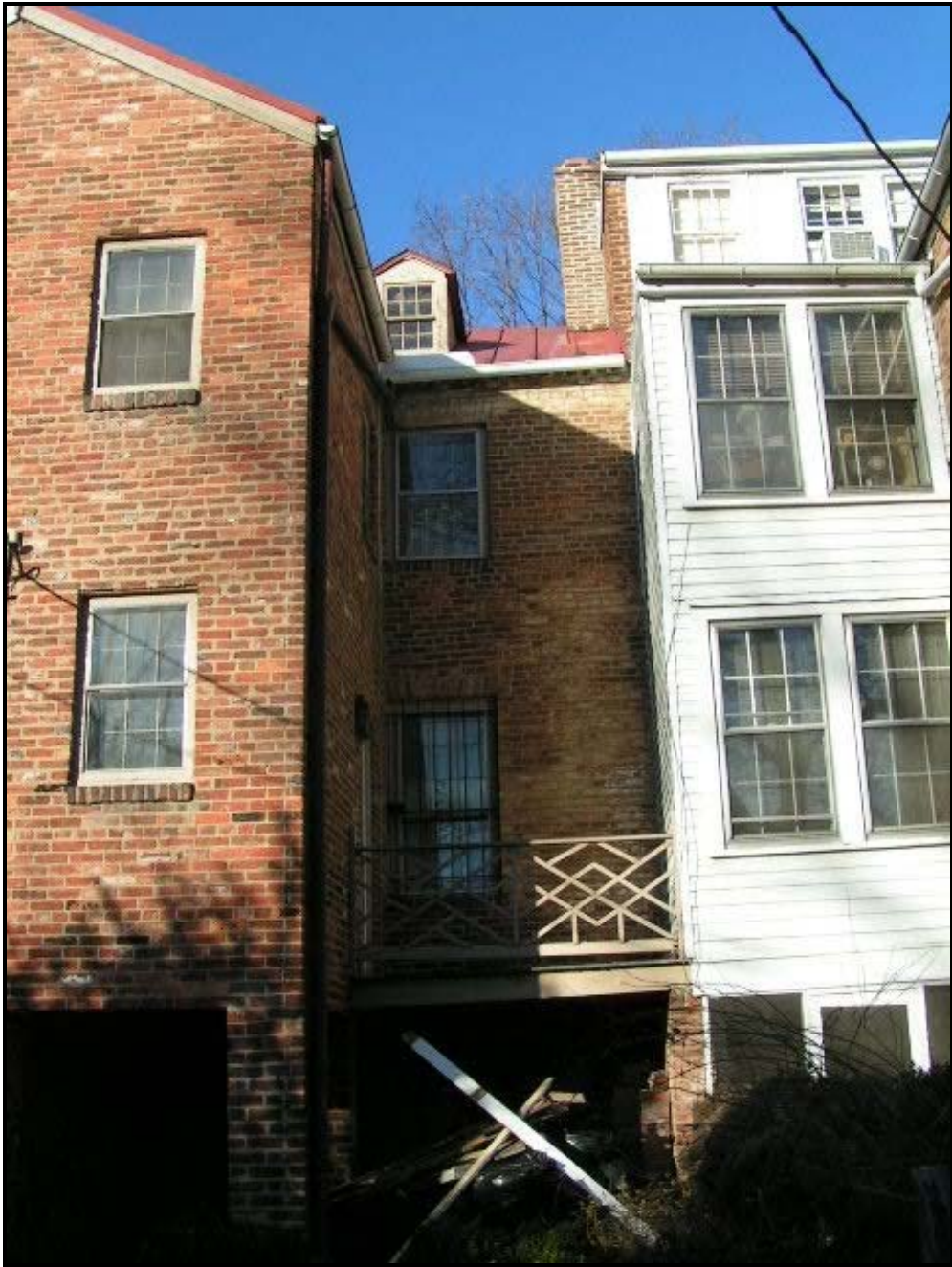
Figure 4: Close up of rear elevation
