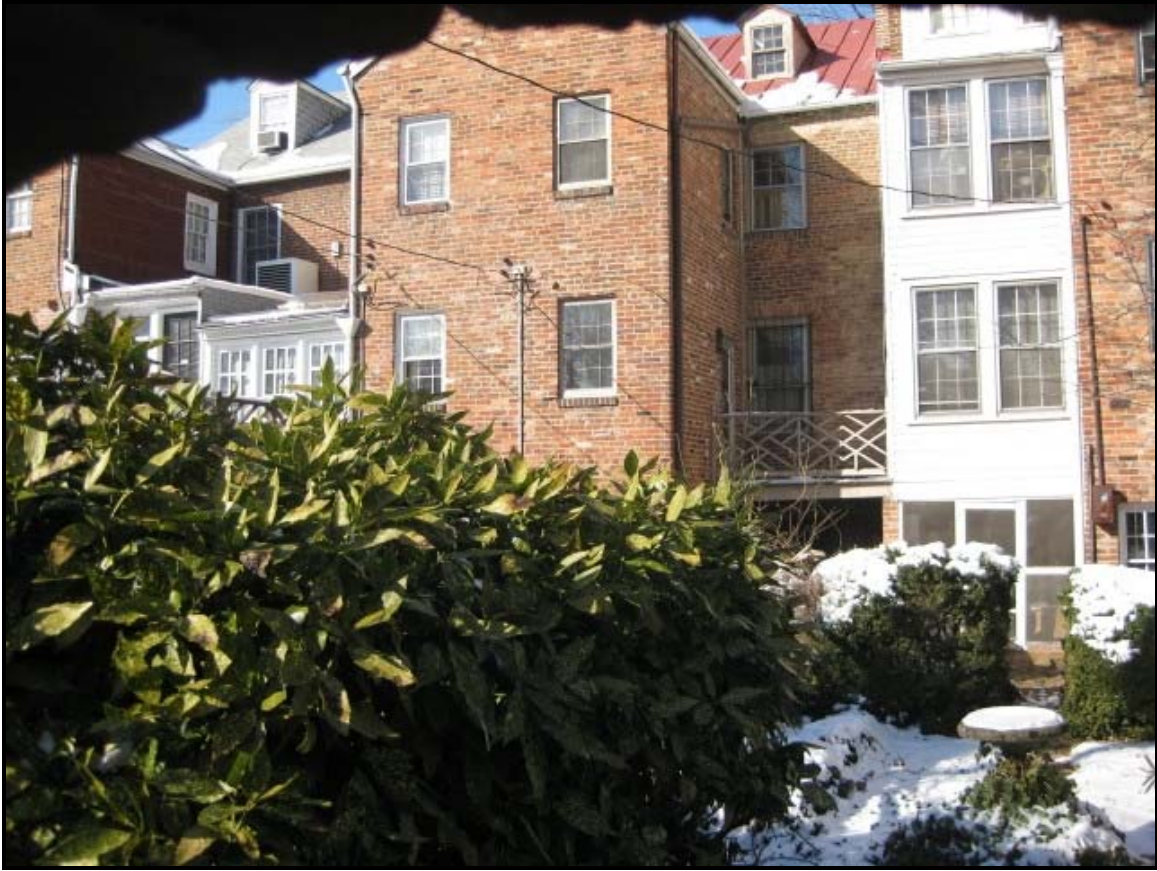
Figure 5: View from alley
