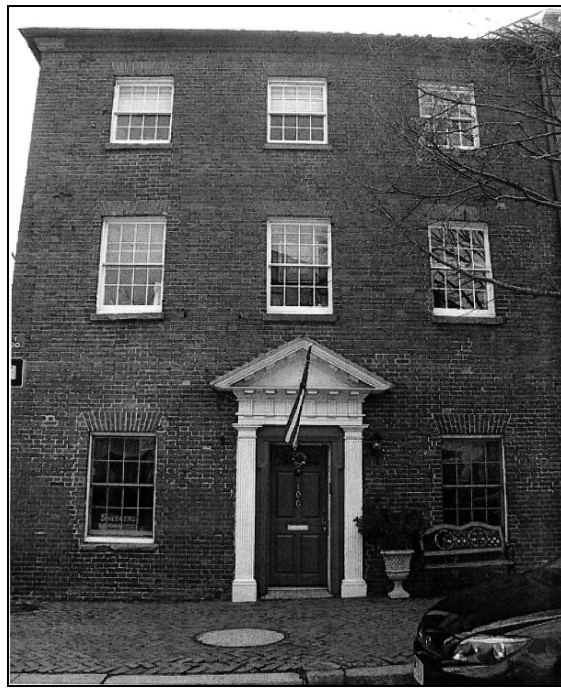
Figure 1. 100 Prince Street: north elevation.
