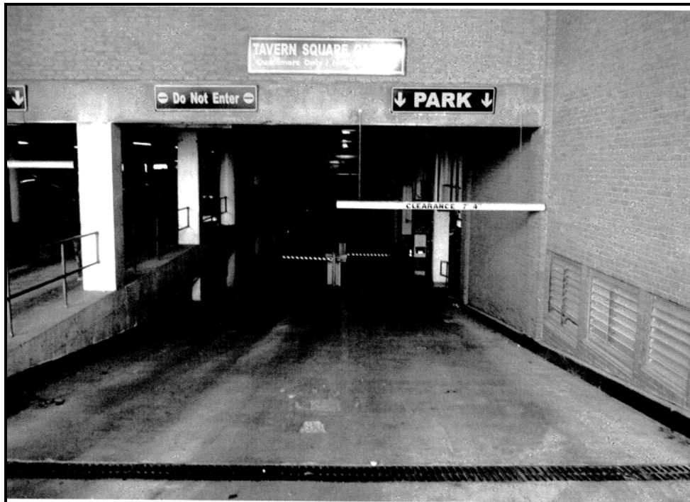
Figure 2: Photograph of Garage Entrance Ramp
