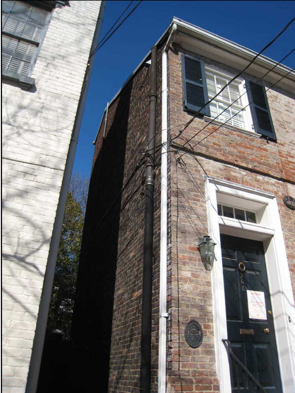
Figure 4: Photo showing side of 208 North Fairfax Street
