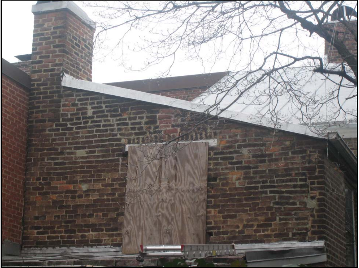
Figure 6: Close up of rear wall to be encapsulated
