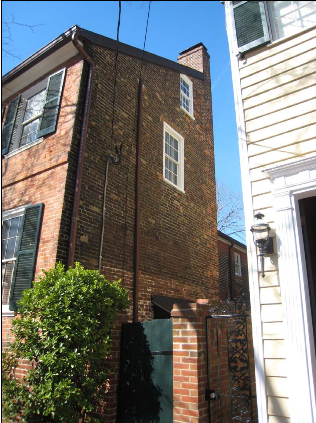
Figure 5: Photo showing front flouder at 210 North Fairfax Street
