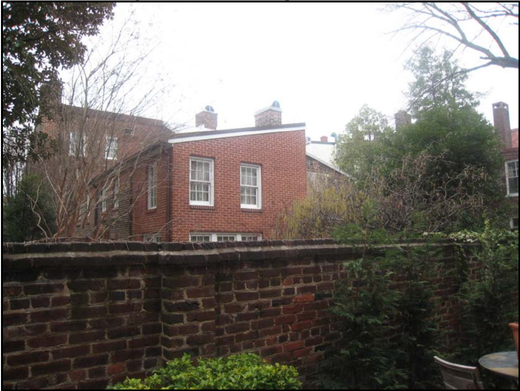
Figure 7: View of 210 North Fairfax Street from pedestrian easement
