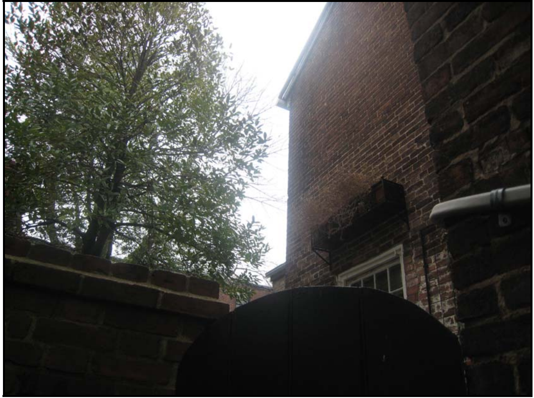
Figure 9: View toward rear from alley next to 208 North Fairfax Street
