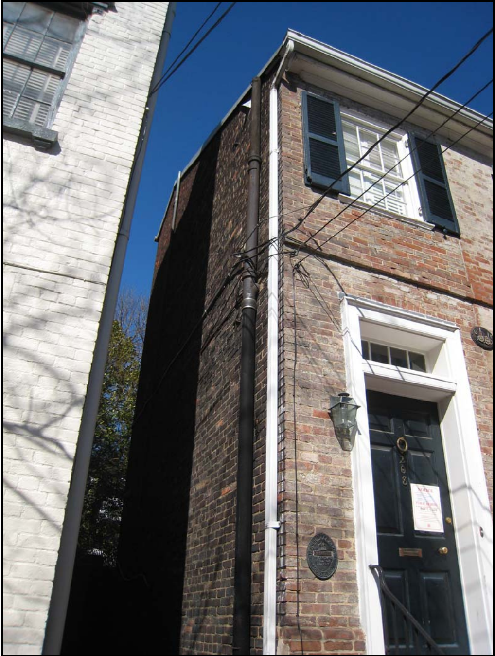
Figure 4: Photo showing front/side of 208 North Fairfax Street
