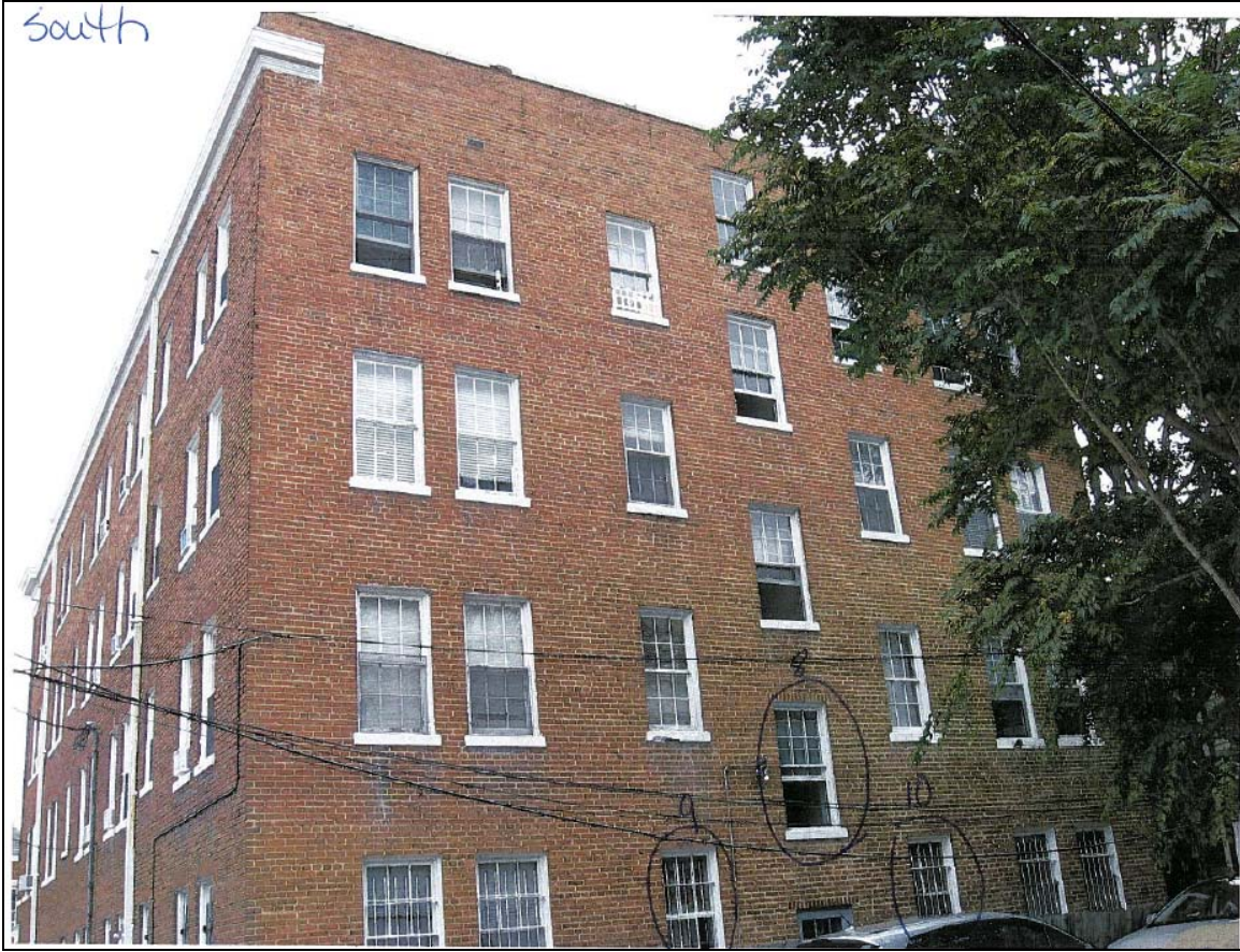
Figure 2. View of rear(south) elevation.
