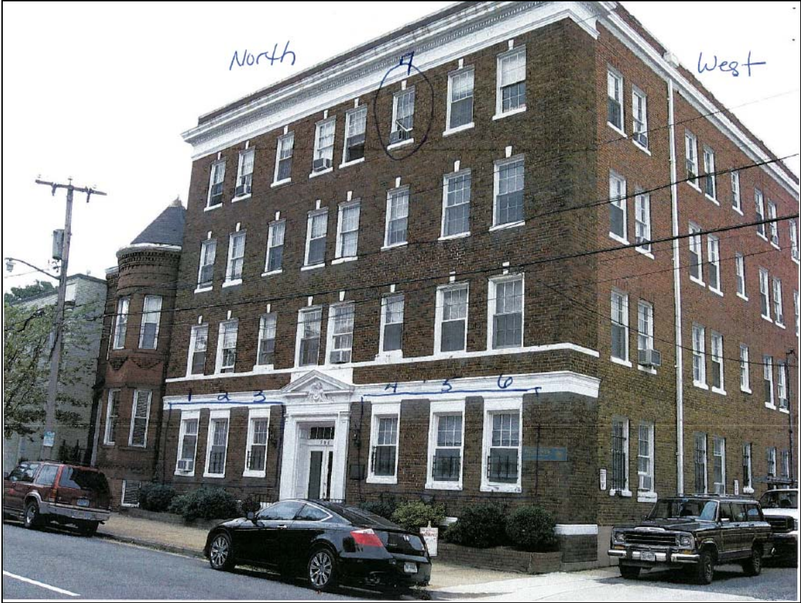
Figure 1. View looking at front and Westside elevation.
