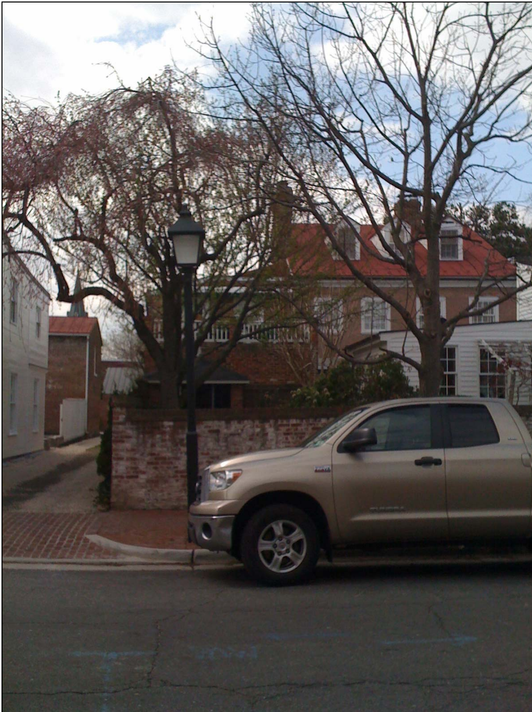
Figure 2: View of Property from Public ROW
