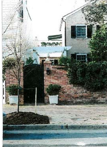
202 Duke Street from the street South Elevation
