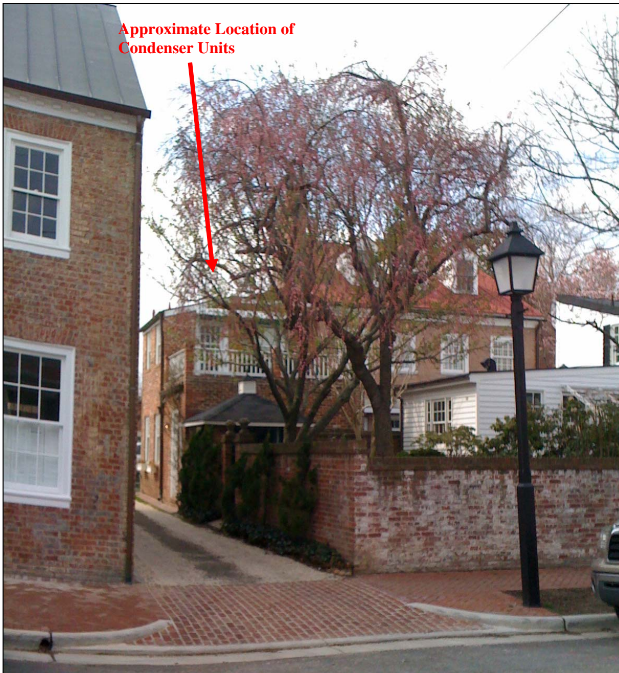
Figure 1: View of Property from Public ROW
