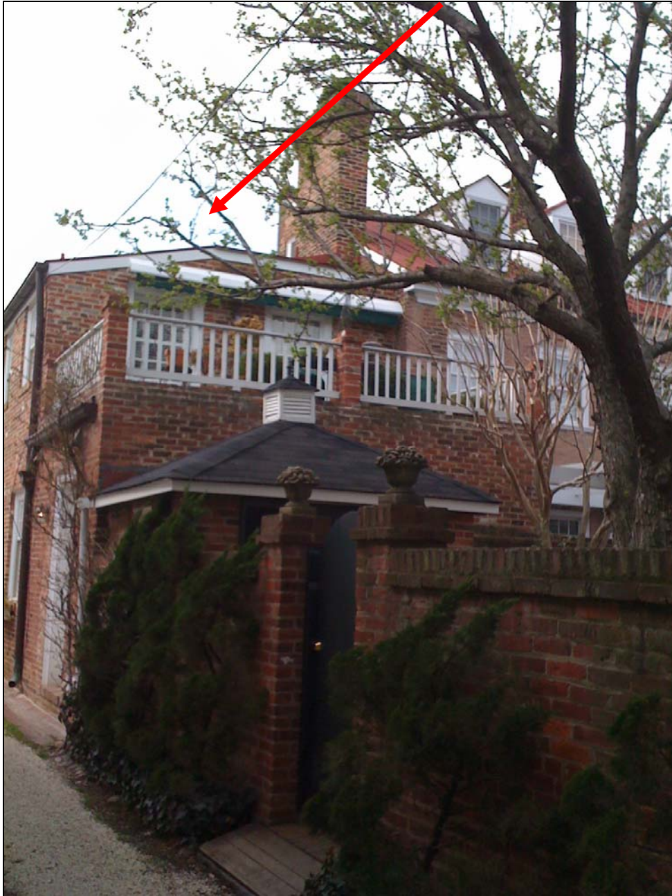
Figure 3: View of Property from Public Alley
