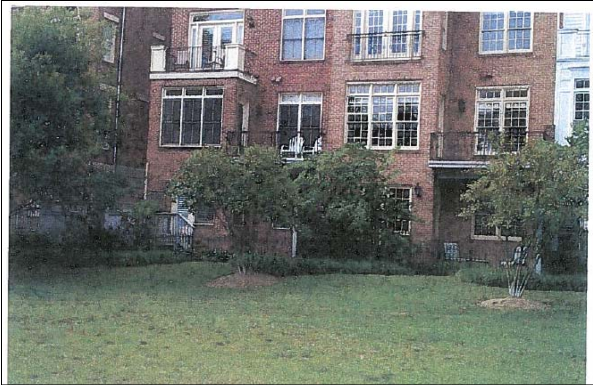
Figure 1. View of the rear (north) elevation of 19 Keith's Lane.
