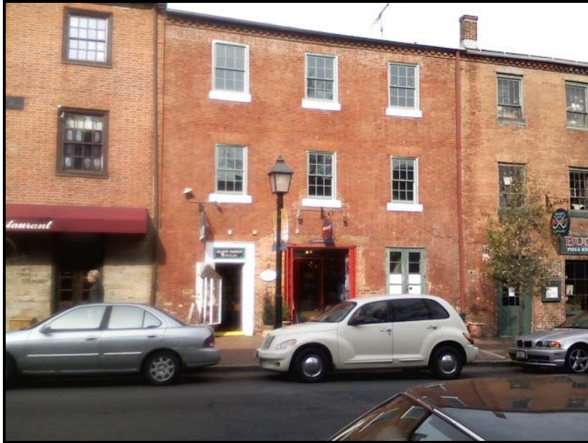
Figure 1 Photograph of the front facade of 113 King Street depicting the 6 replacement windows.
