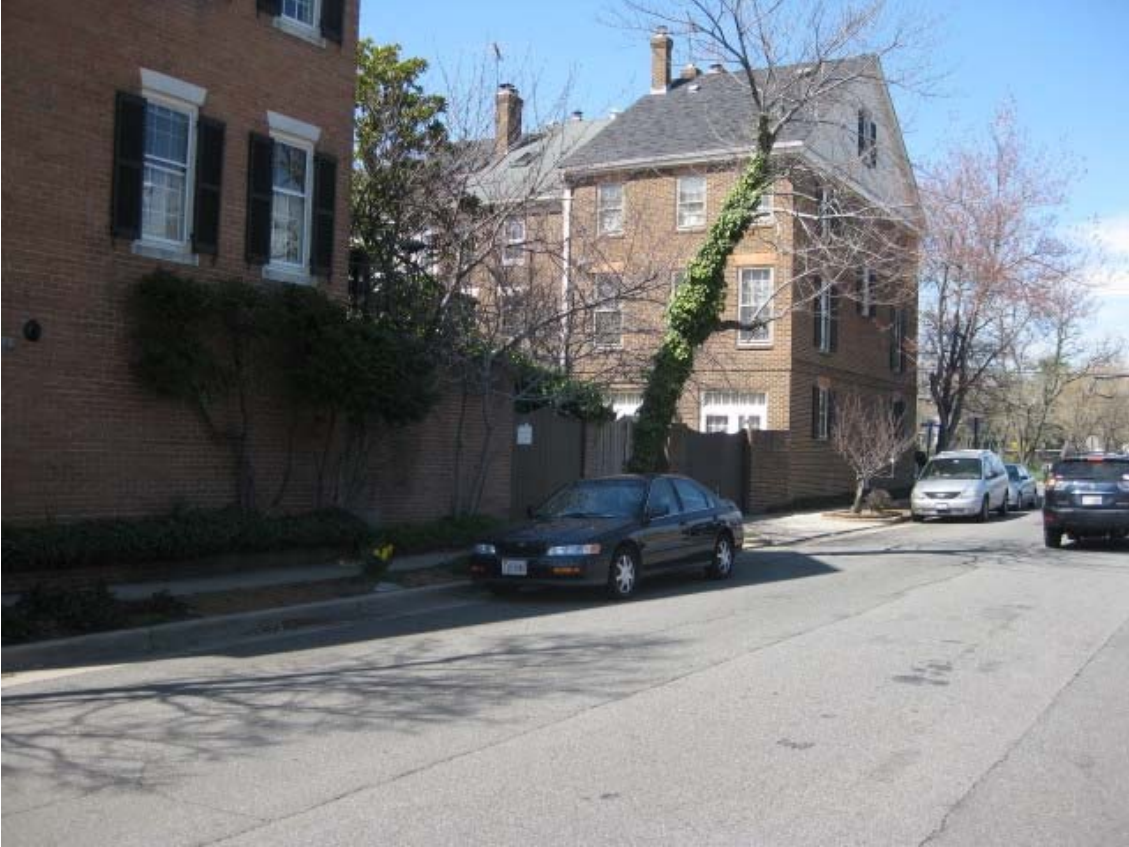
Figure 5. Photo of rear elevation (2nd house in from street)
