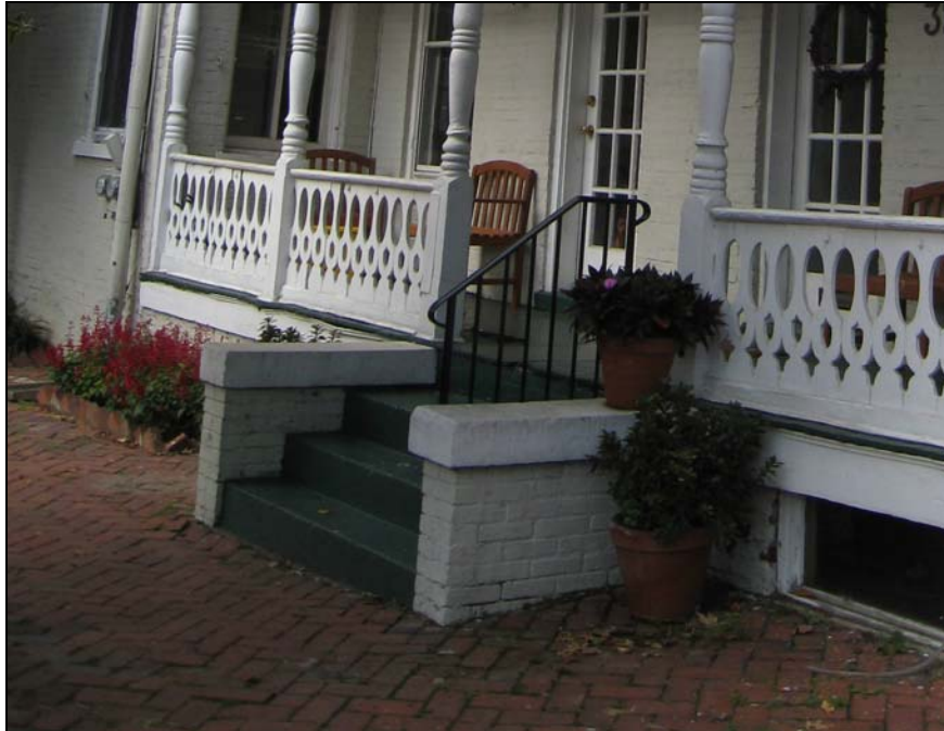
Figure 6. Detail of stoop.
