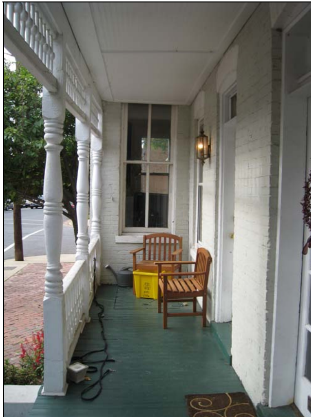
Figure 5. Detail of first floor of porch.
