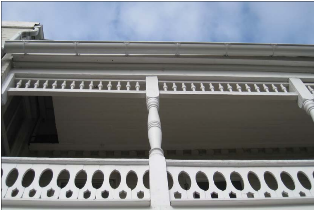
Figure 7. View of roof box from second story porch ceiling.
