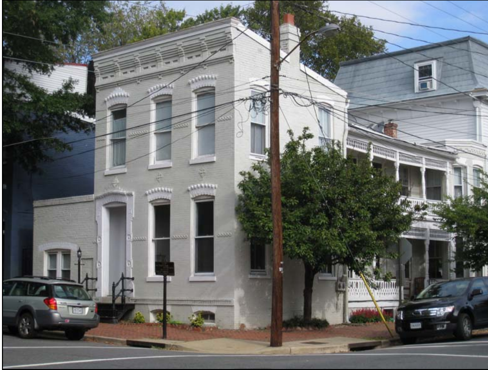
Figure 2. Oblique view of 501 Wolfe Street, existing conditions.
