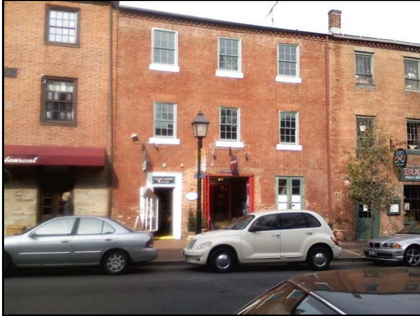
Figure 1 Photograph of the front facade of 113 King Street depicting the 6 replacement windows.
