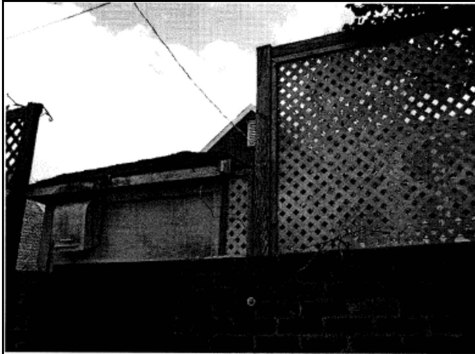
Figure 12: View of 911 South St. Asaph Street from behind 913 South St. Asaph Street
