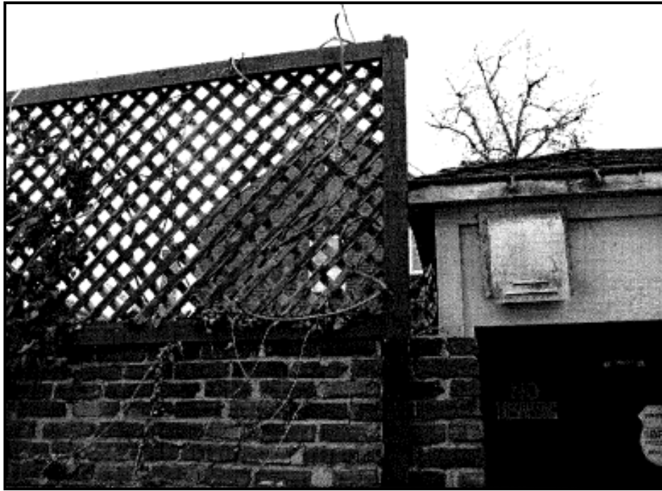
Figure 11: View from the property line shared by 911 and 913 South St. Asaph Street
