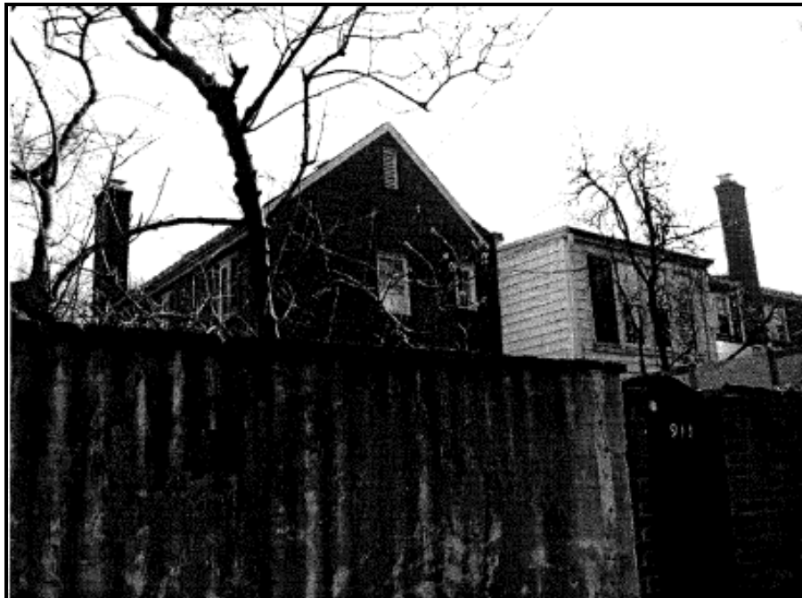
Figure 8: View from behind 909 South St. Asaph Street
