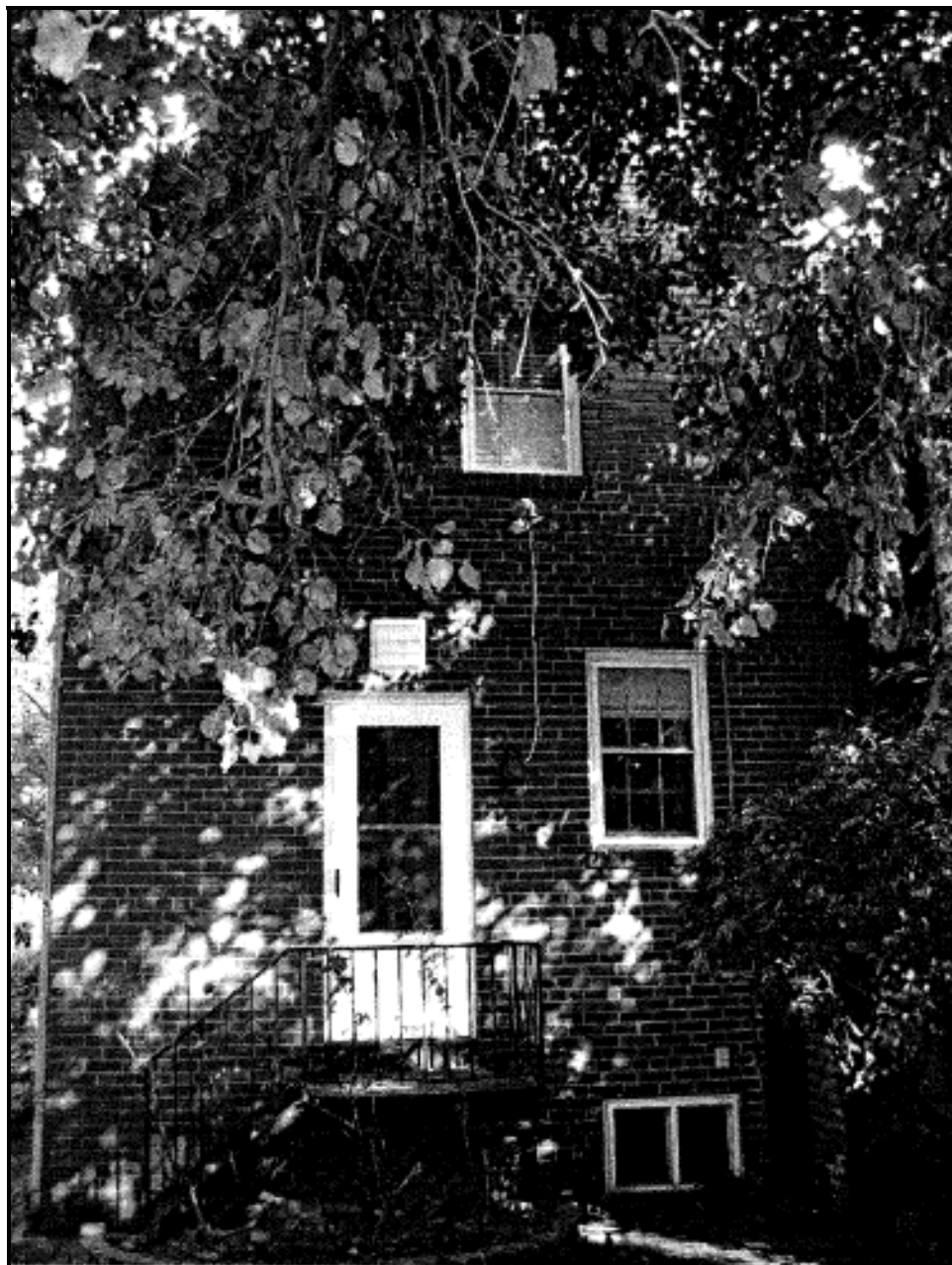
Figure 4: View of the Rear (west side) of 911 South St. Asaph Street from the courtyard
