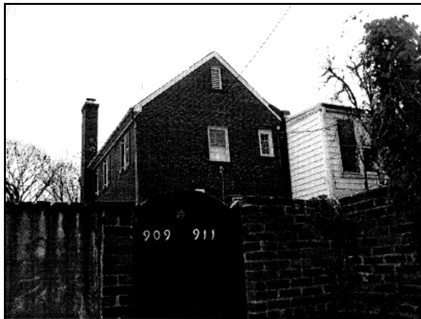
Figure 9: View from the property line shared by 909 and 911 South St. Asaph Street
