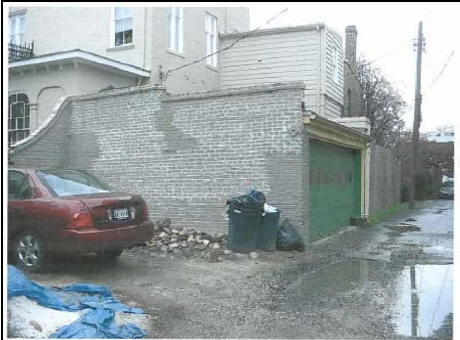
Existing Garage Door and Parking Space (6/4/09 photo)
