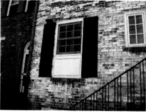
832 S Lee St – Replacement windows
