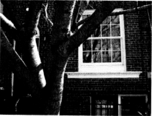
810 S Lee St – Replacement windows
