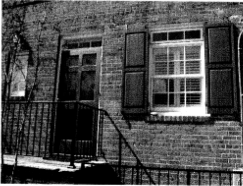
809 S Lee St – Replacement windows
