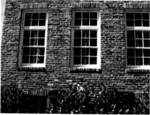
833 S Lee St – New Windows - Clad
