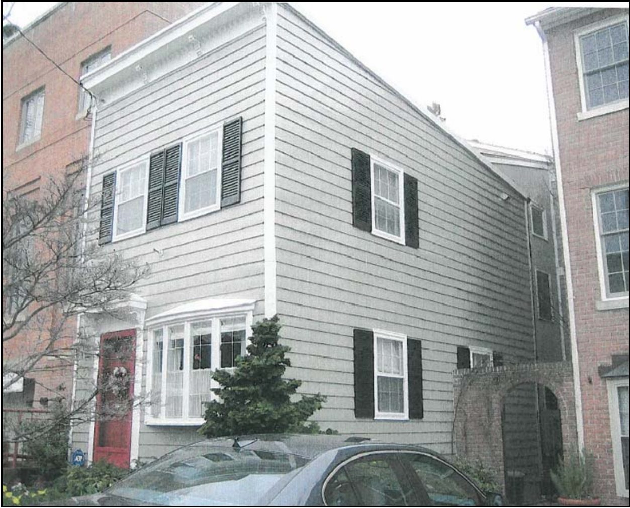
Figure 1. Front and side (east) elevation.
