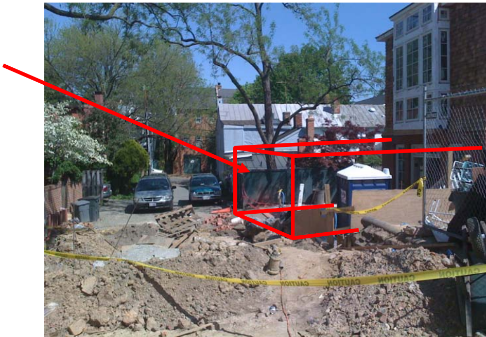
Figure 4. Photo of existing conditions. View from City Parking Lot.
