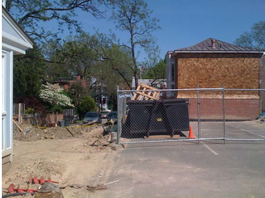
Figure 4. Photo of existing conditions. View from City Parking Lot.
