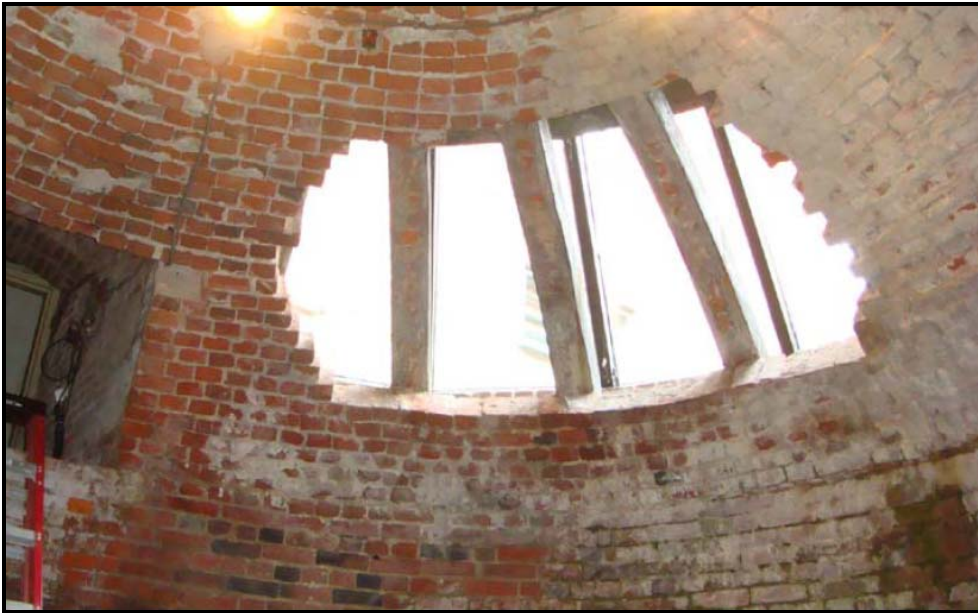
Figure 3: Interior of Ice Well
