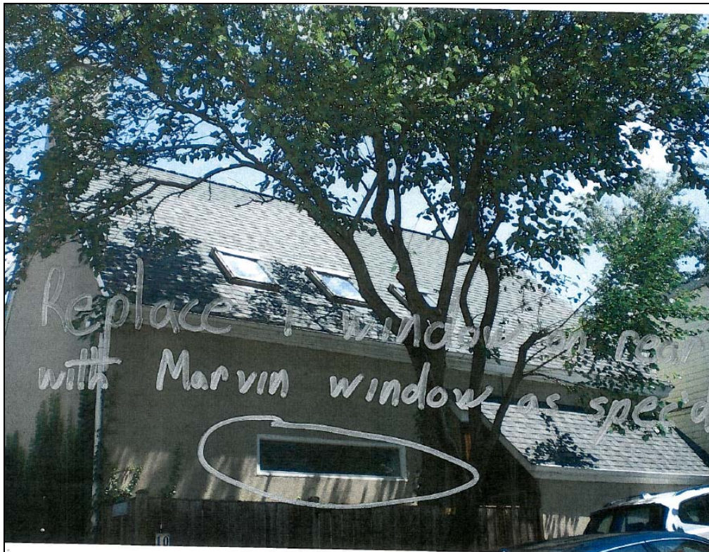
Figure 2. South elevation, 10 Irving Court, indicating window proposed for replacement.
