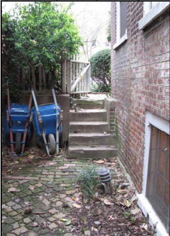
Figure 7: Existing Side Elevation looking toward Lee Street and side yard gate
