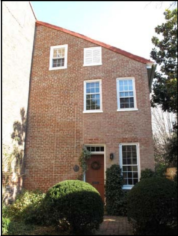
Figure 2: Front facade (west elevation) of 220 South Lee Street
