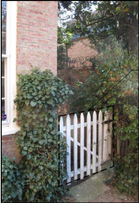
Figure 6: Existing side yard gate to be replaced
