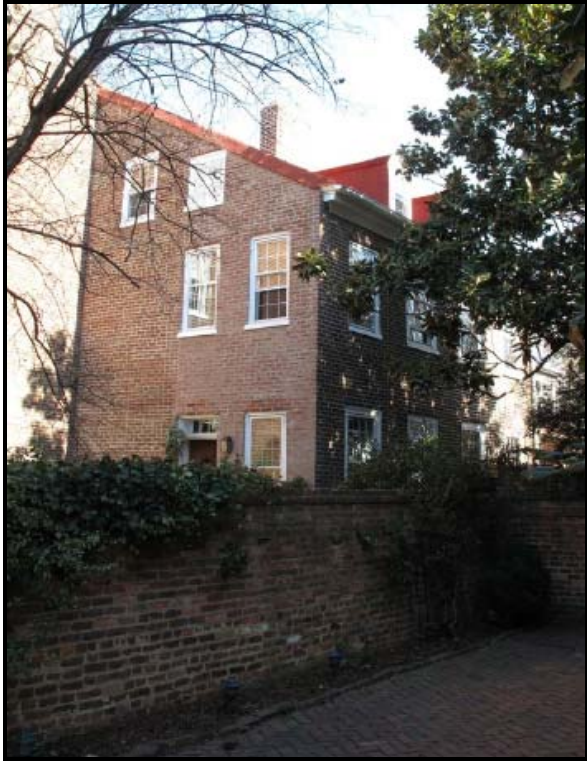
Figure 4: Close up of front (west) /side (south) elevation
