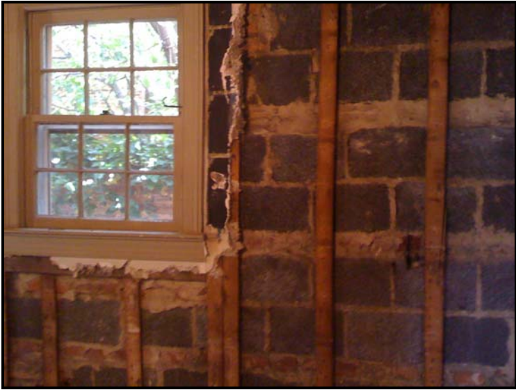
Figure 16: Interior View of Mid-20 th century brick addition
