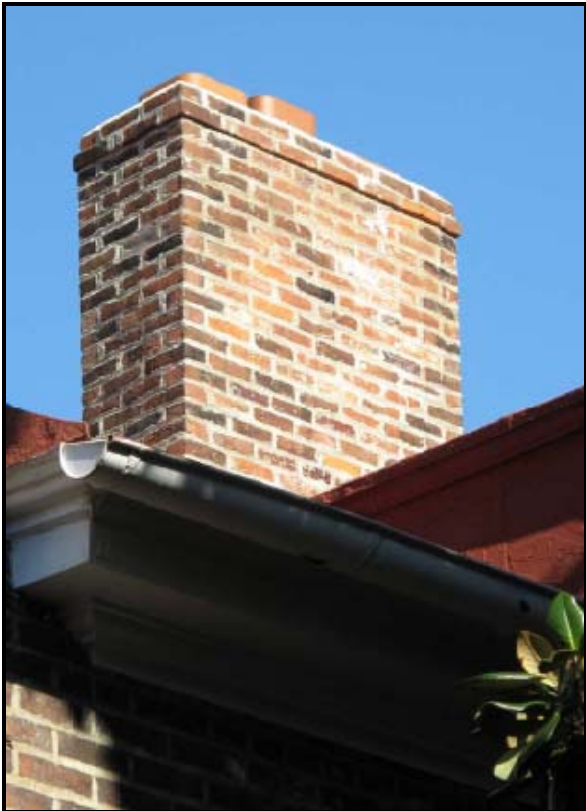
Figure 13: View of Chimney
