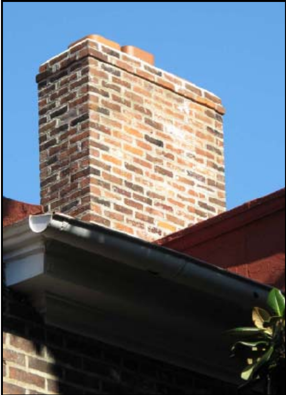
Figure 13: View of Chimney
