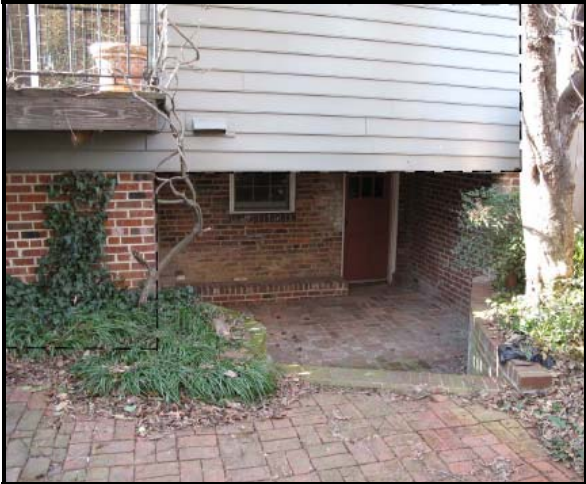
Figure 12: View of Existing Basement Level
