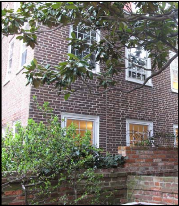
Figure 8: Existing south elevation
