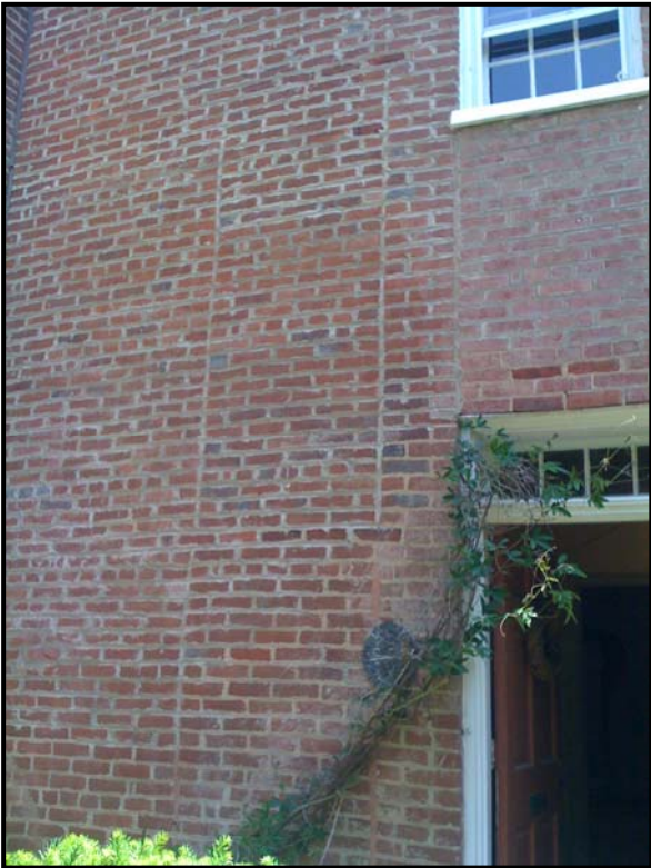
Figure 15: View of Front Elevation & "Visual Documentation" of previous window
