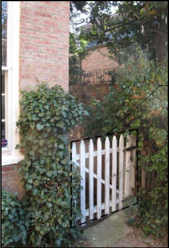
Figure 6: Existing side yard gate to be replaced
