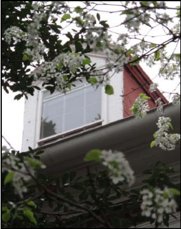
Figure 14: View of Existing Dormer
