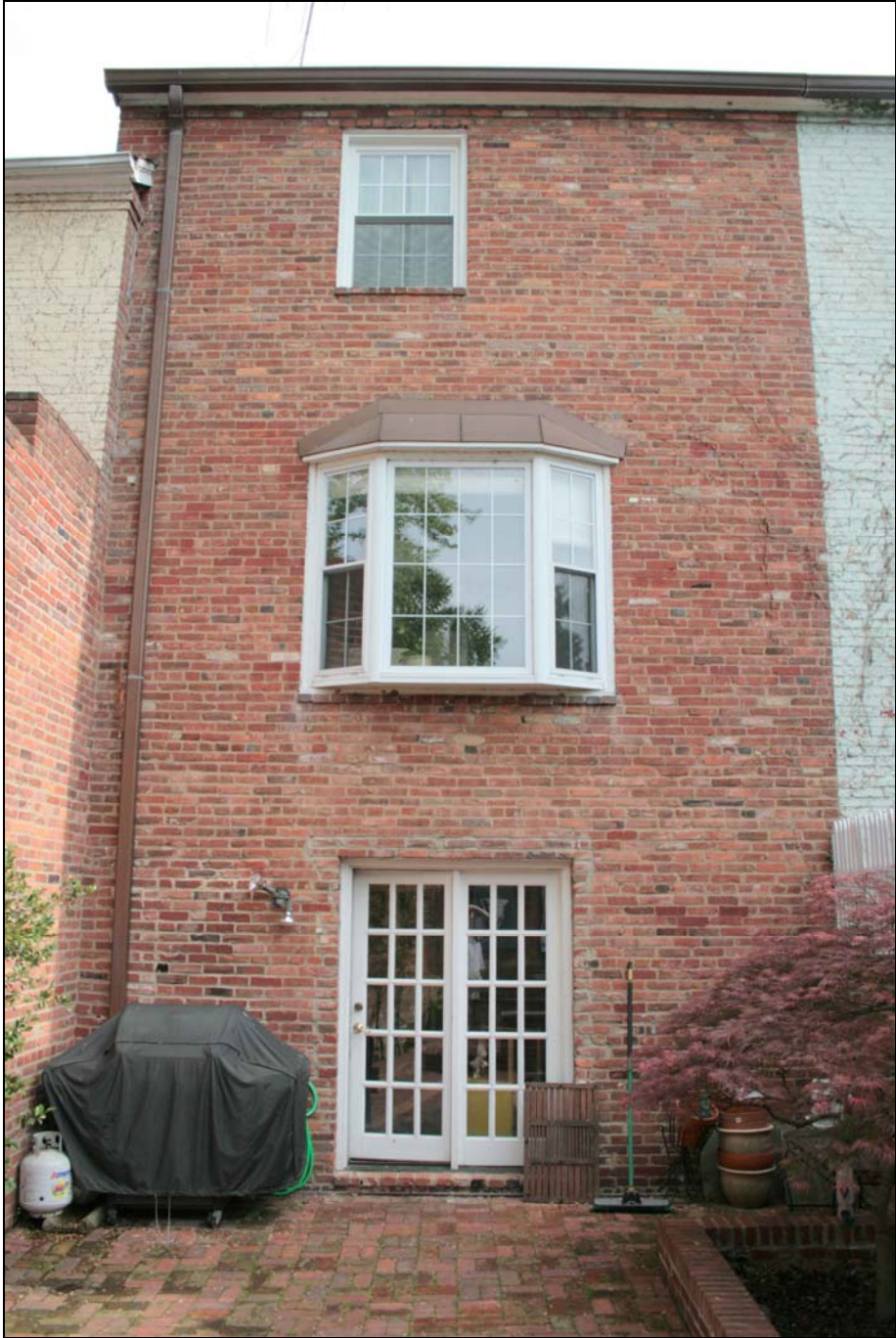
Figure 2. Rear (south) elevation of 404 Jefferson Street. Top window is visible from public right-of-way.
