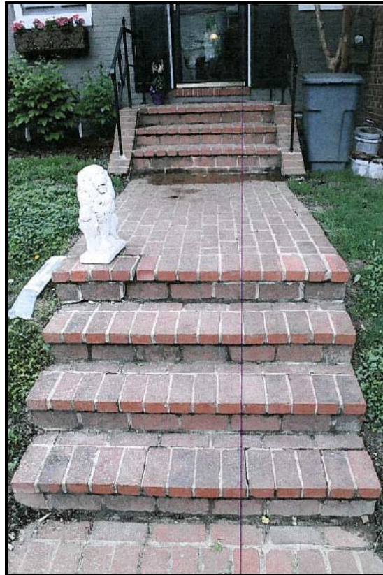
Figure 5: Photograph of Existing Steps
