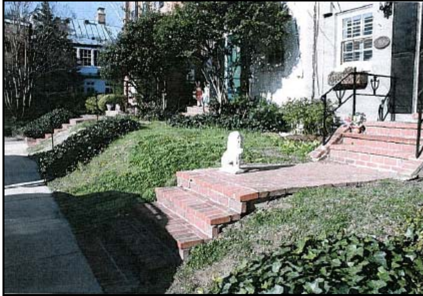
Figure 6: Photograph of Existing Steps
