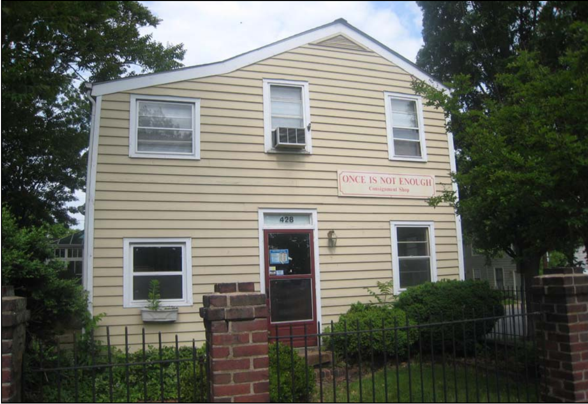
Figure 3. Front (east) elevation.
