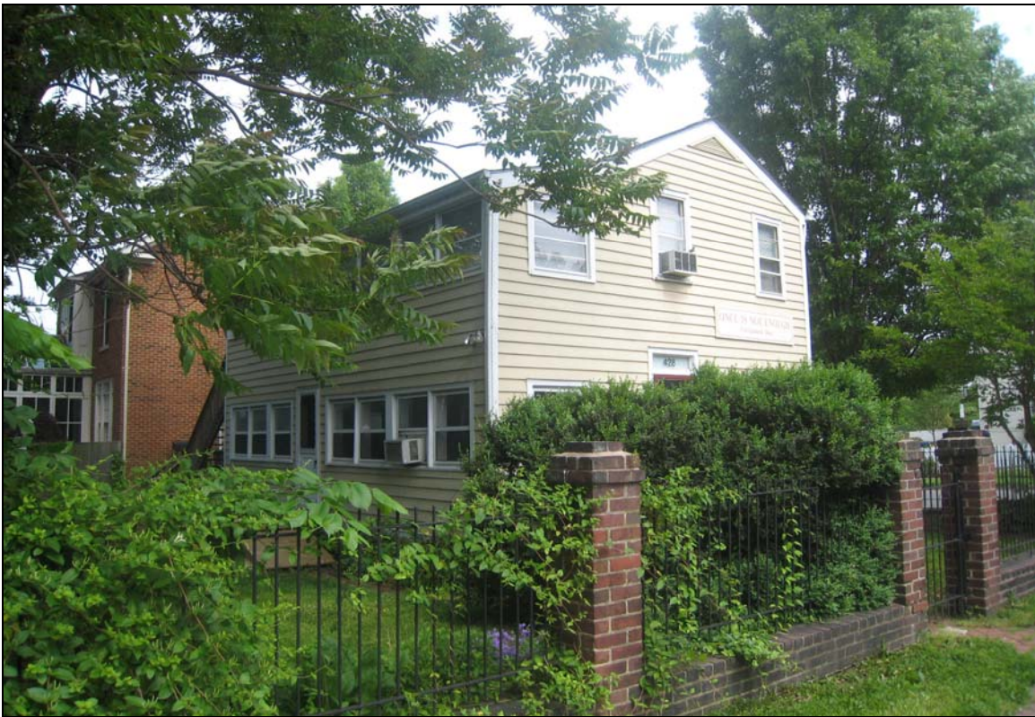
Figure 4. Oblique view showing enclosed porch on side (south) elevation.
