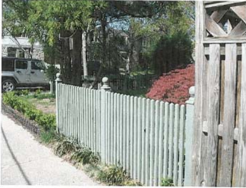
Fence on Michigan Avenue
