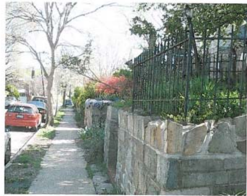
Michigan Avenue retaining wall and fence
