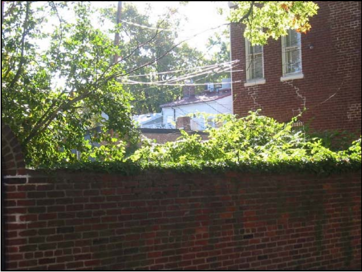
Figure 4. Rear of house as seen from St. Asaph Street.
