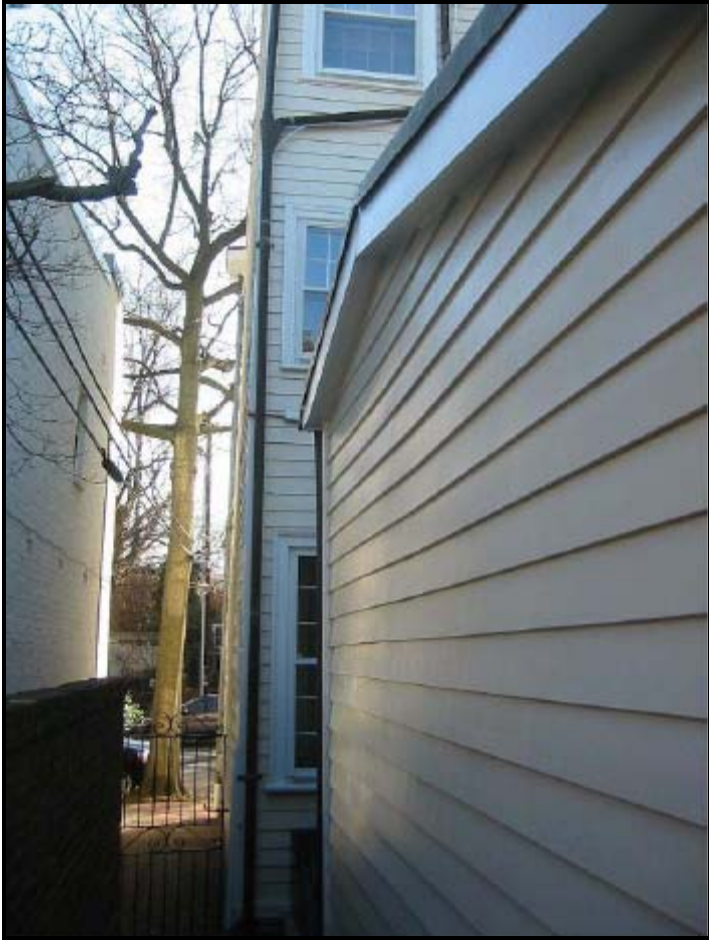
Figure 5. Existing rear elevation and one story addition.
