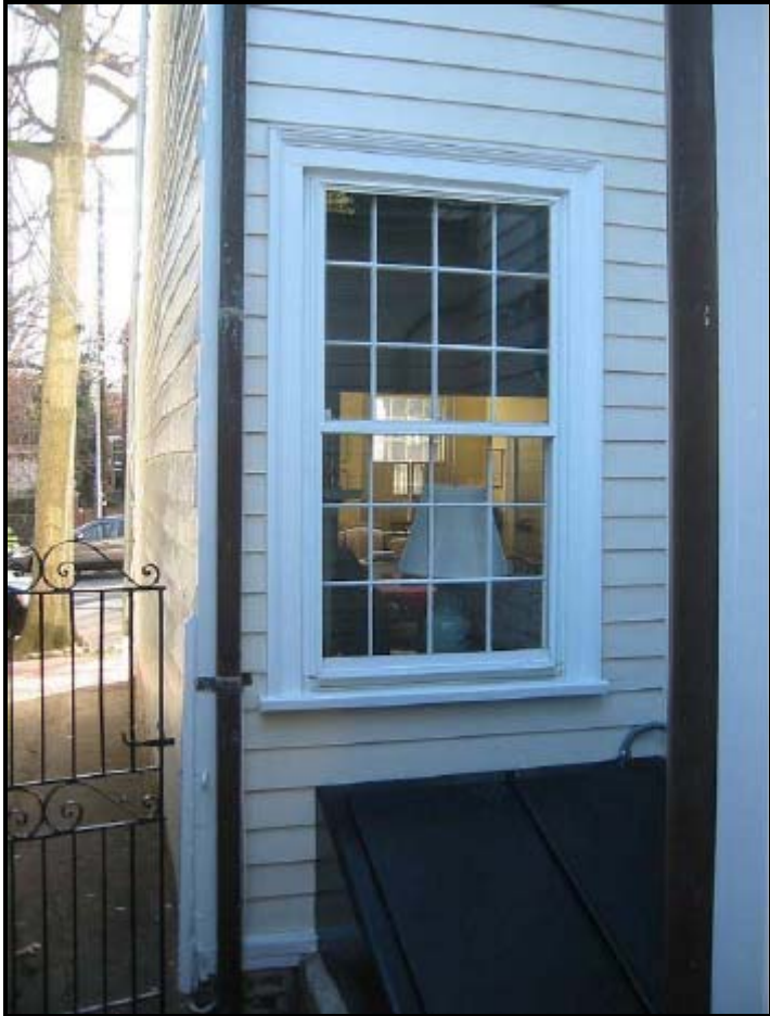
Figure 6. Existing 12 over 12 window on main portion of the house.
