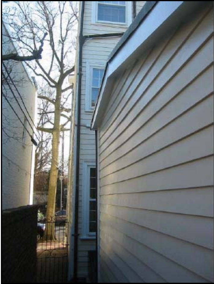
Figure 5. Existing rear elevation and one story addition.
