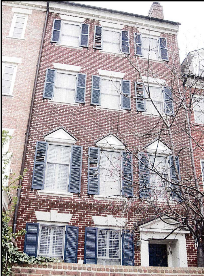
Figure 1. Photograph of the existing front facade.
