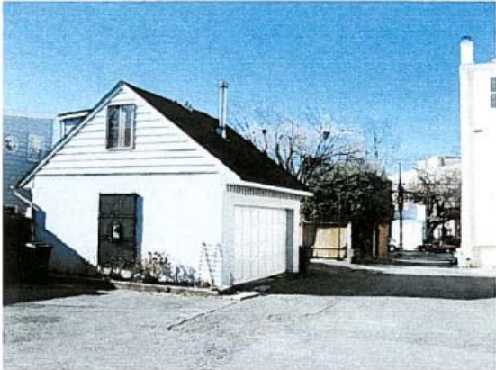
View of 1217 Prince St. garage taken from rear alley
