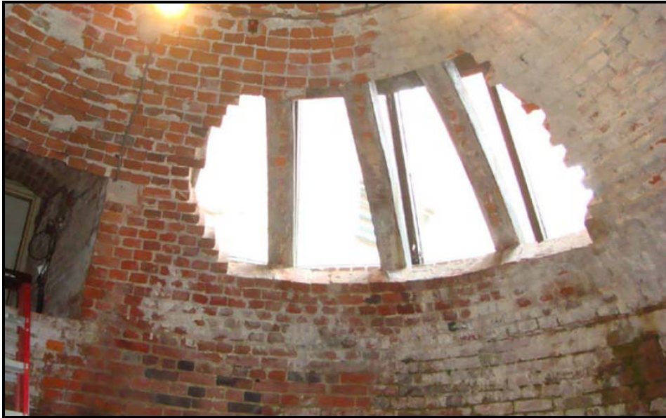
Figure 3: Interior of Ice Well
