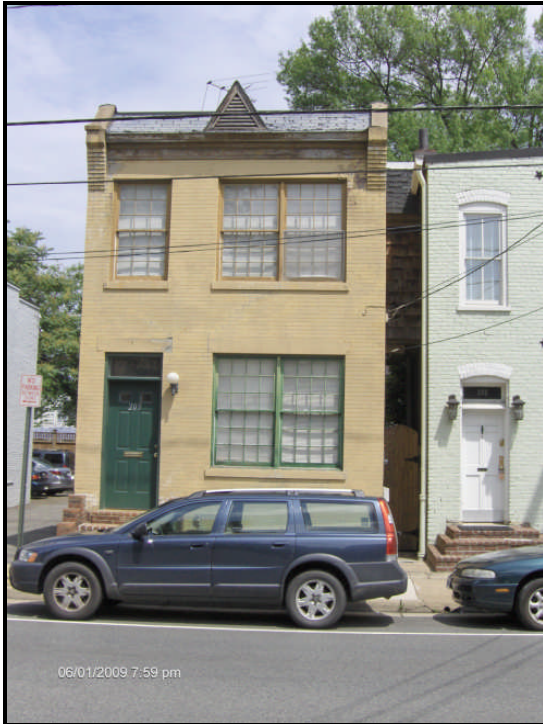
Figure 4. Photograph of front façade
