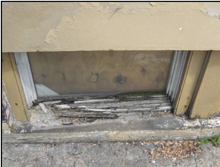
Figure 6. Detail photograph of basement level window
