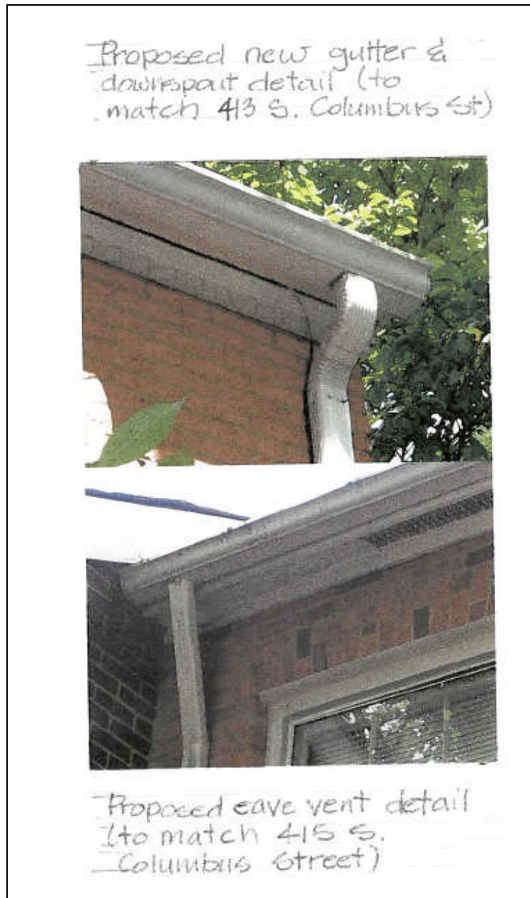
Figure 7. Examples of gutter repairs.
