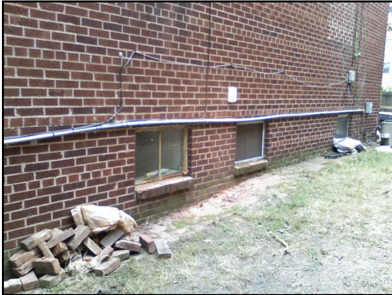
Figure 3. Photograph of basement windows on north elevation
