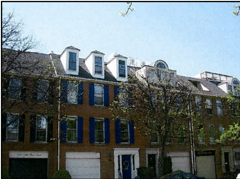
Figure 2. Photograph depicting roof decks of neighboring properties.
