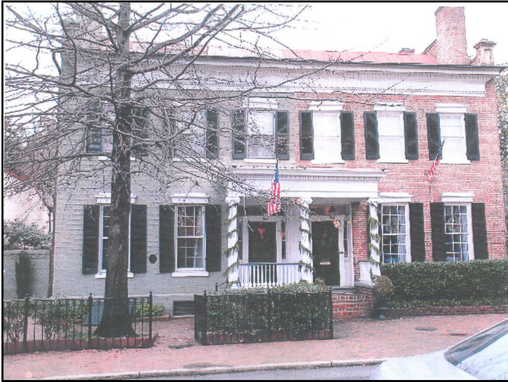
Figure 2: Front (east) elevation.
