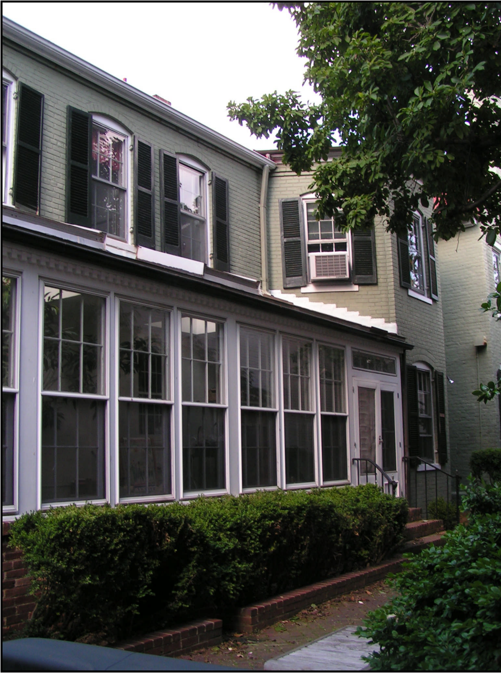
Figure 4: Photo of enclosed side porch prior to construction.
