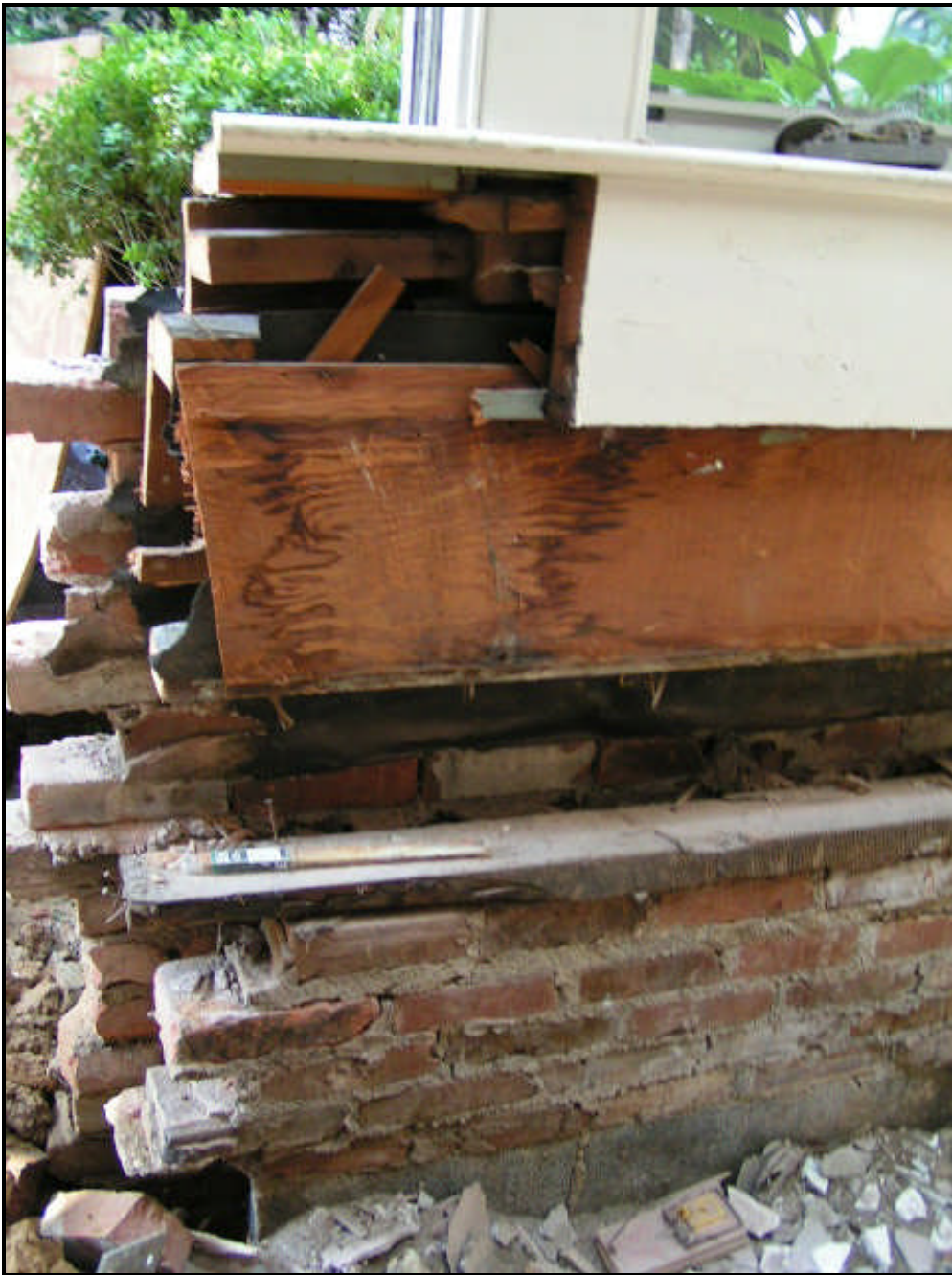
Figure 7: Close up of south wall of enclosed porch.
