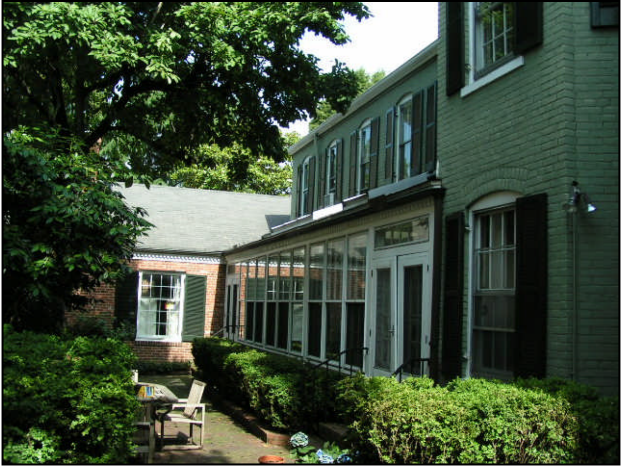
Figure 3: Photo of enclosed side porch prior to construction.
