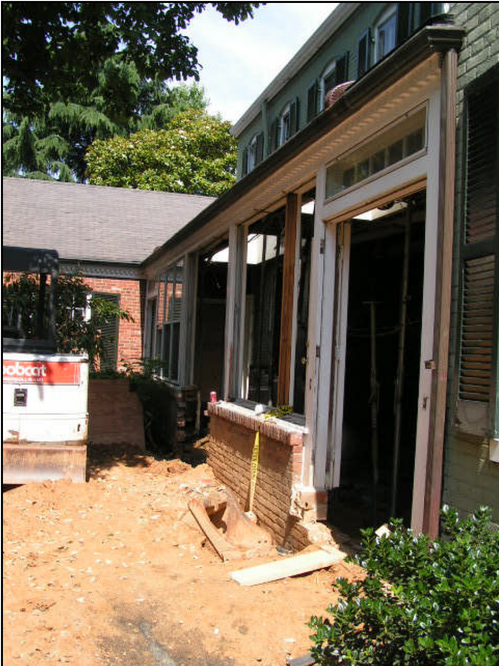
Figure 5: Existing photo of enclosed side porch.
