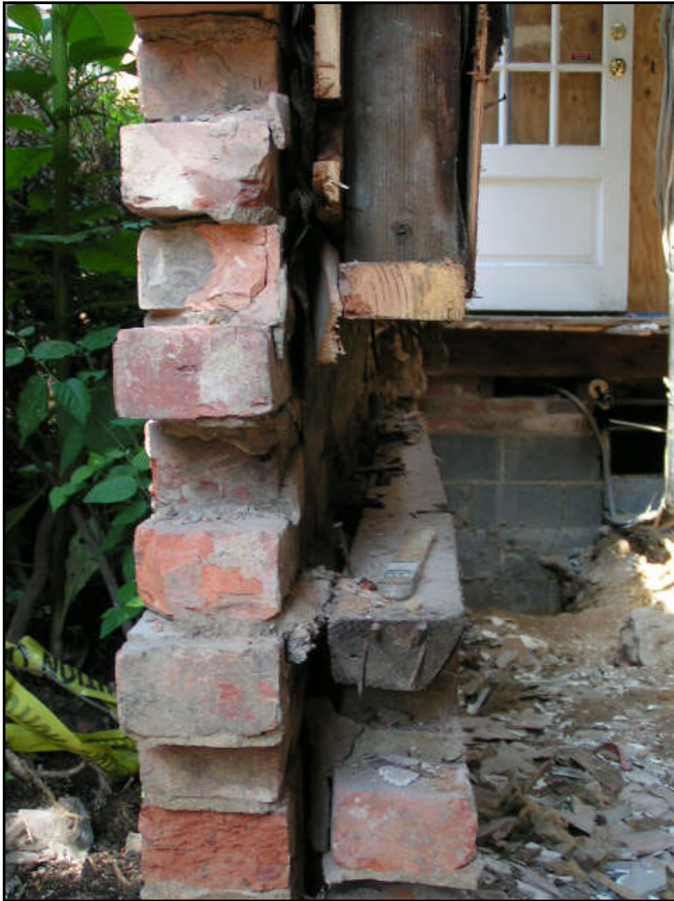
Figure 6: Close up of south wall of enclosed porch.
