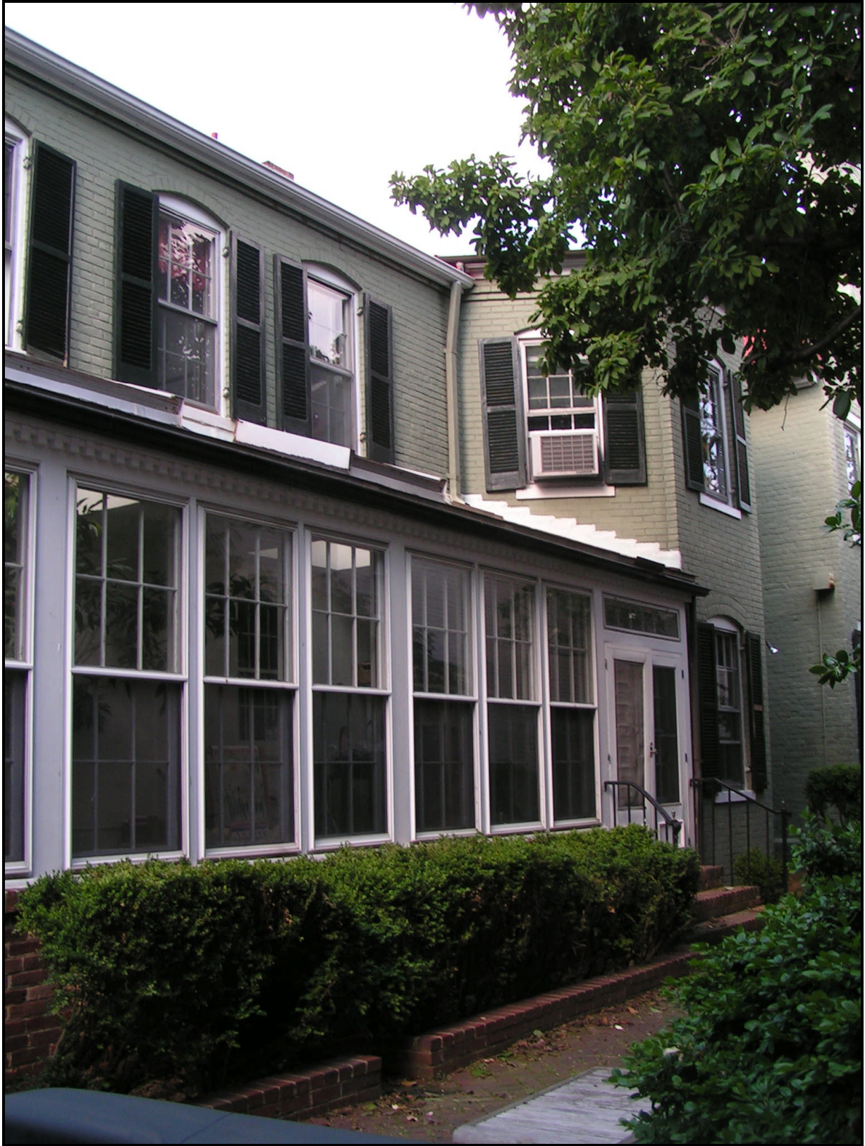
Figure 4: Photo of south elevation of porch prior to construction.
