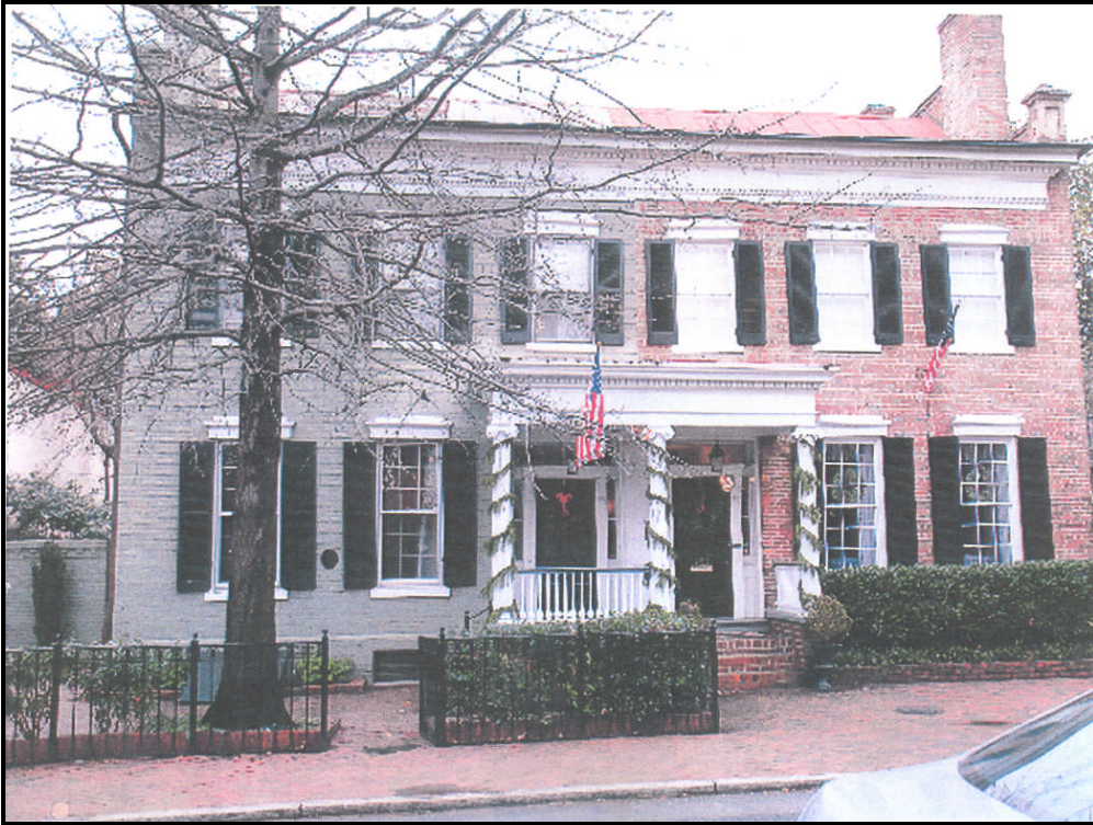
Figure 2: Existing front/east facade.
