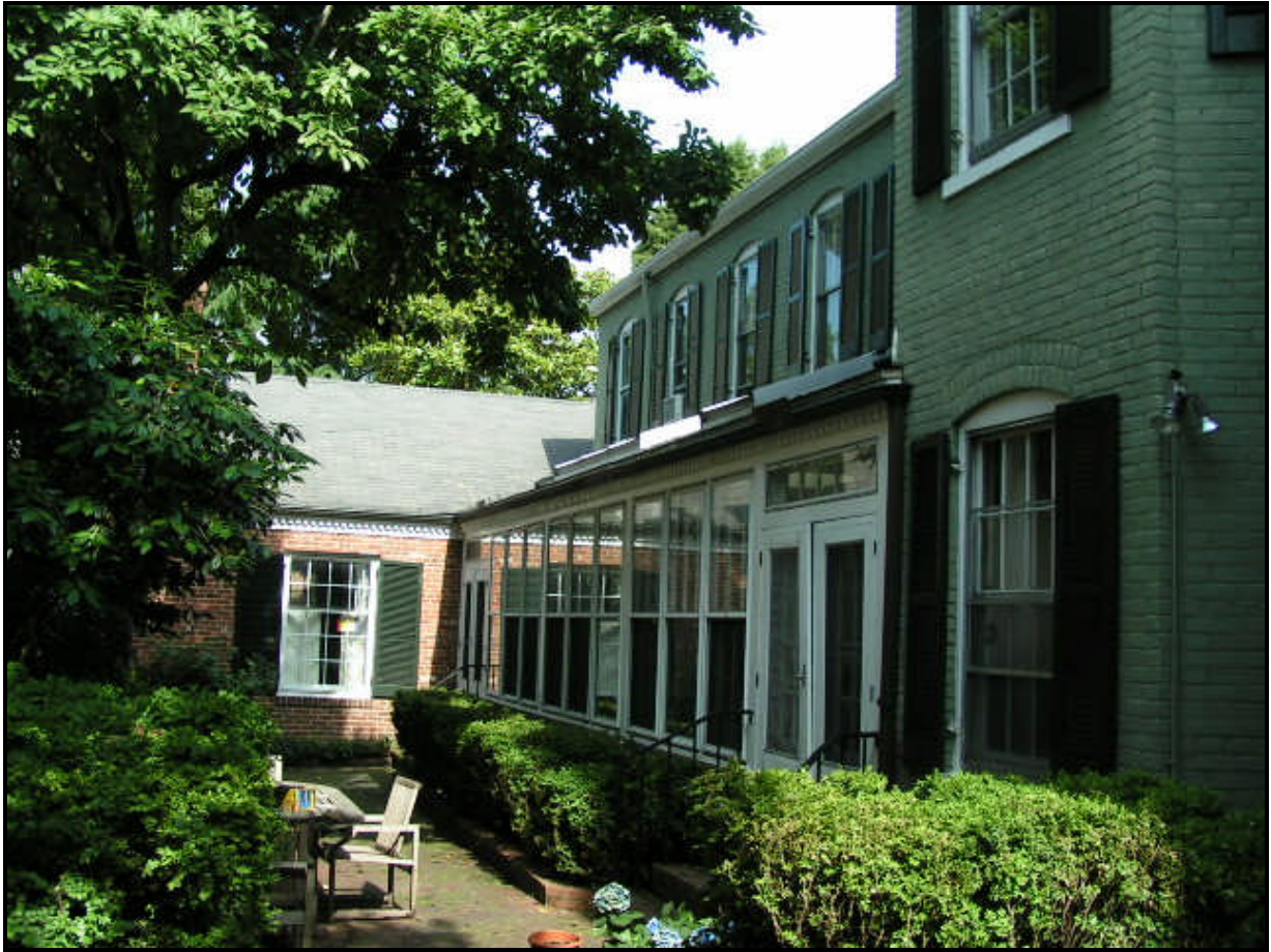
Figure 3: South and east elevations of house prior to start of construction.
