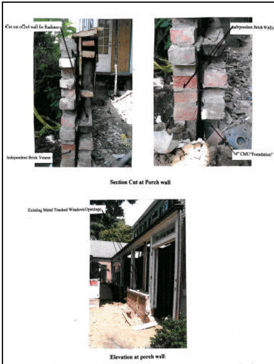
Figure 5: Photos of porch during construction.
