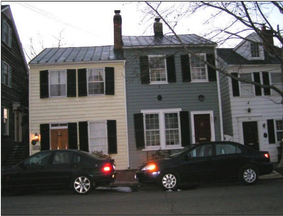
Figure 1. Front (east) elevation of 607 South Fairfax Street (left).
